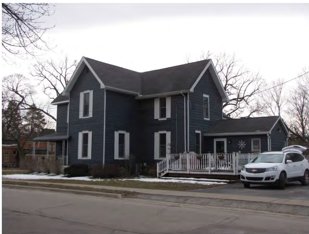
Rogers South 102_Looking Southeast
