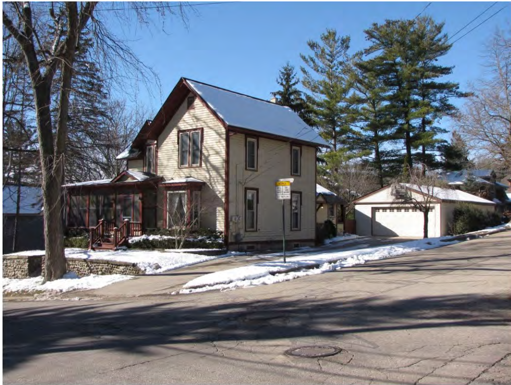
Rogers North 231, Garage_Looking West
