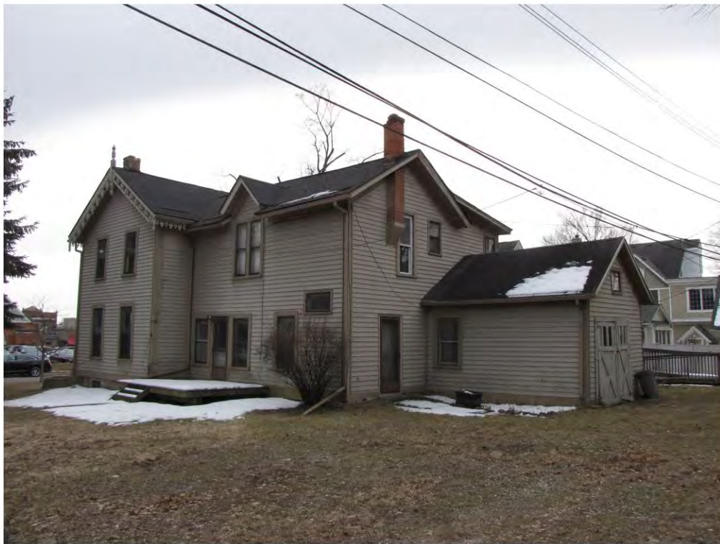
Wing North 129_Looking Southeast
