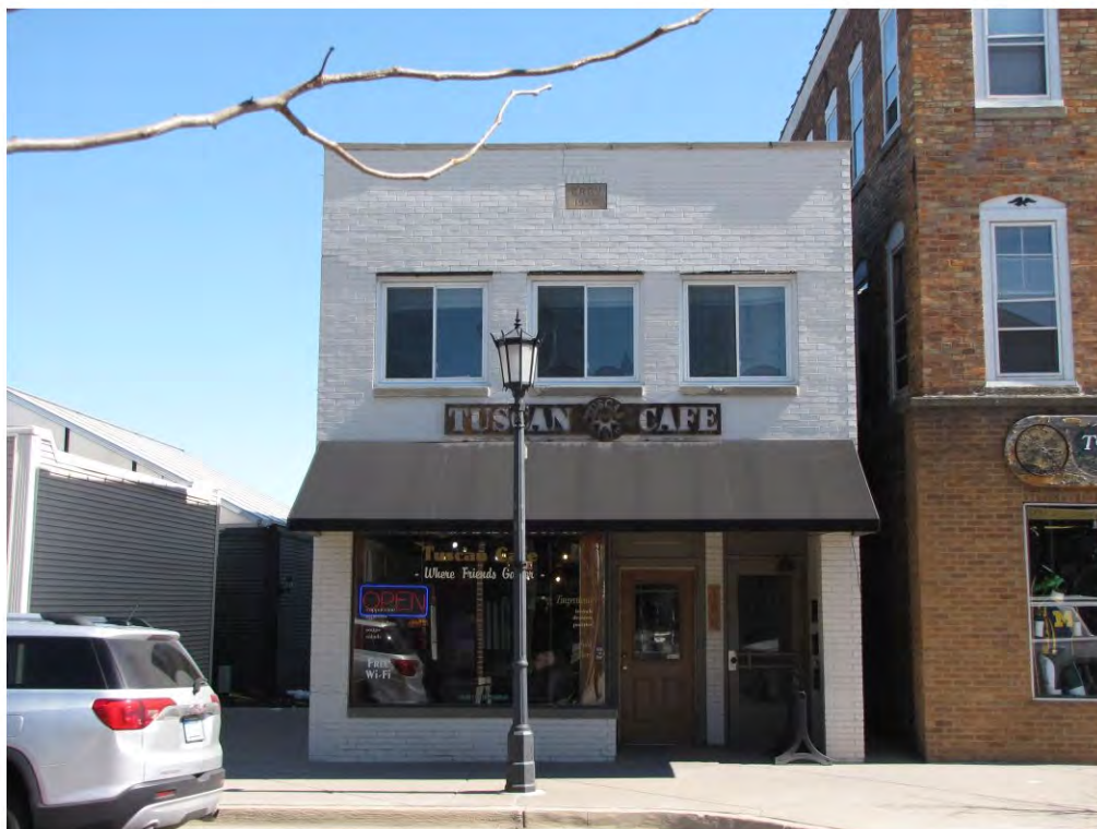
Center North 150_Looking East
