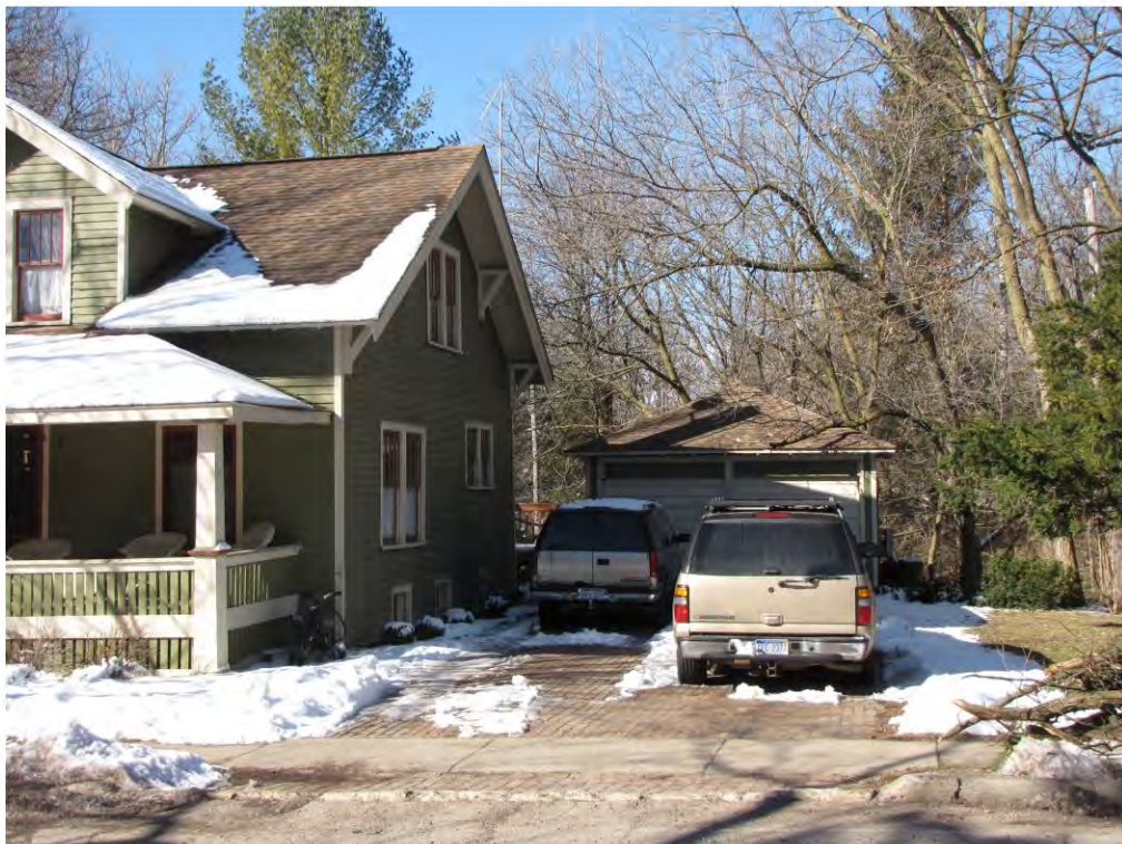
Rogers North 131, Garage_Looking West
