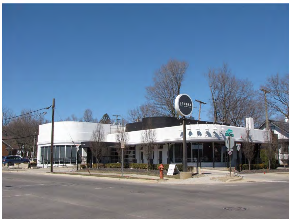
Main West 202_Looking Northwest
