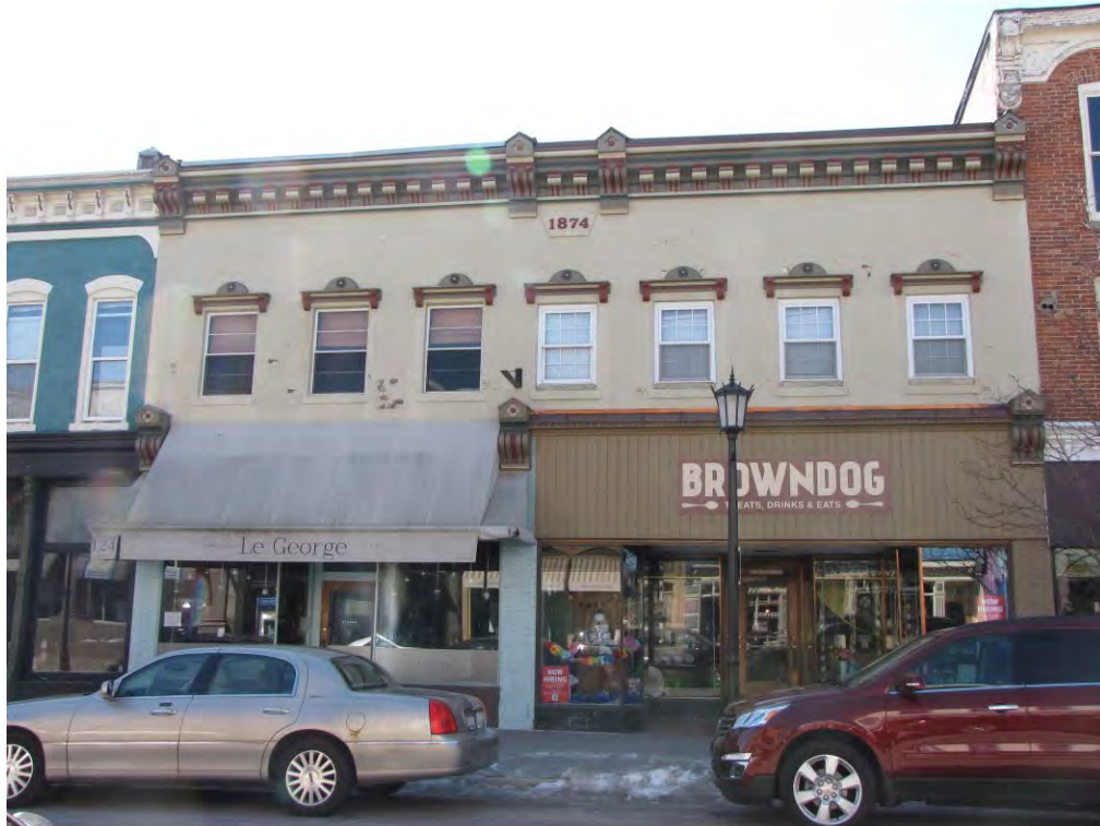
Main East 120-124_Looking South
