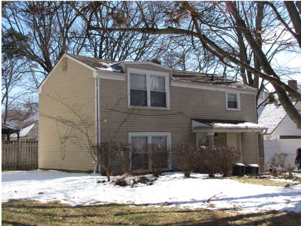
Rogers North 114-116_Looking Southeast
