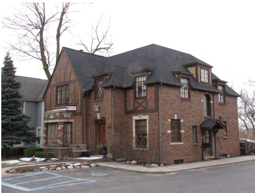
Main East 324_Looking Southeast
