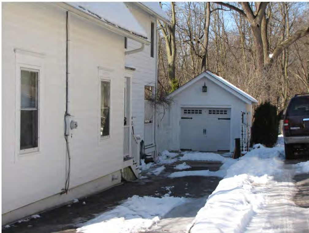
Rogers North 207, Garage_Looking West
