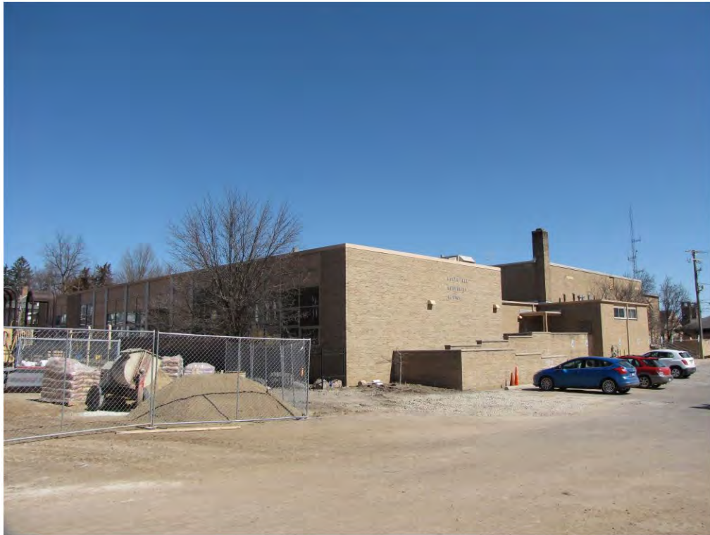
Main West 303_Looking Northeast
