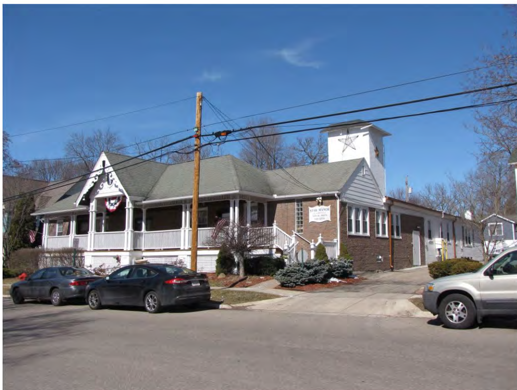
Main West 520_Looking Northwest
