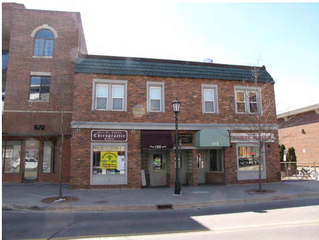
Main West 109-113_Looking South
