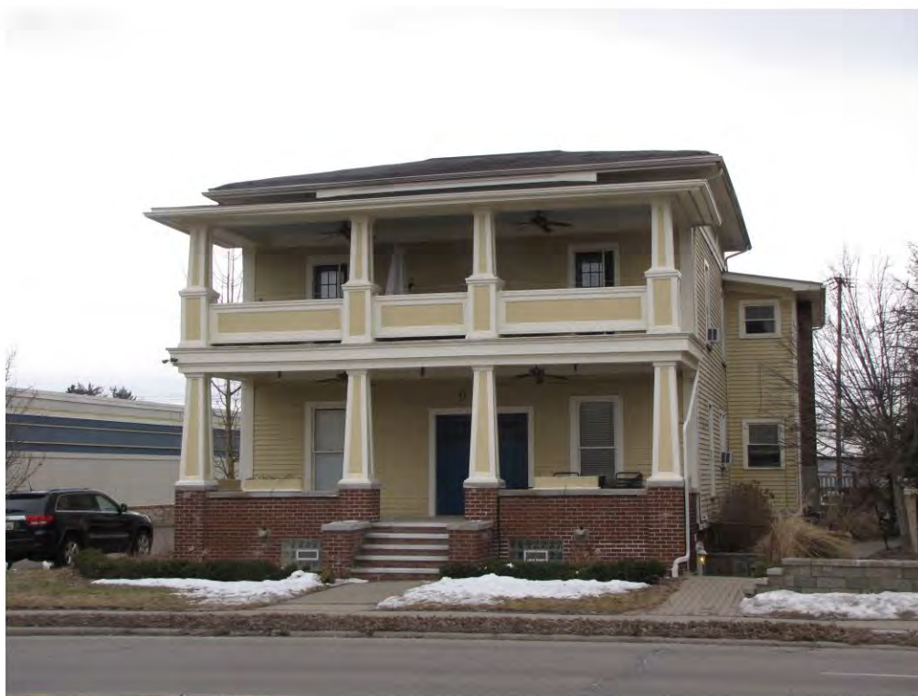
Main East 450_Looking Southeast
