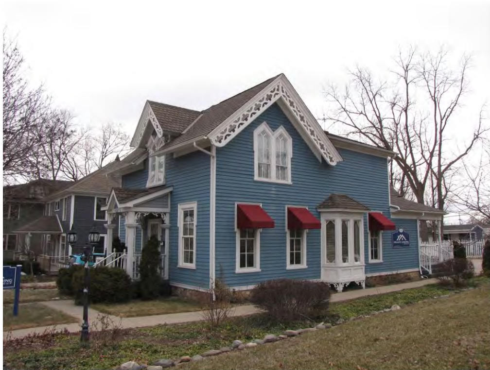
Main East 410_Looking Southeast
