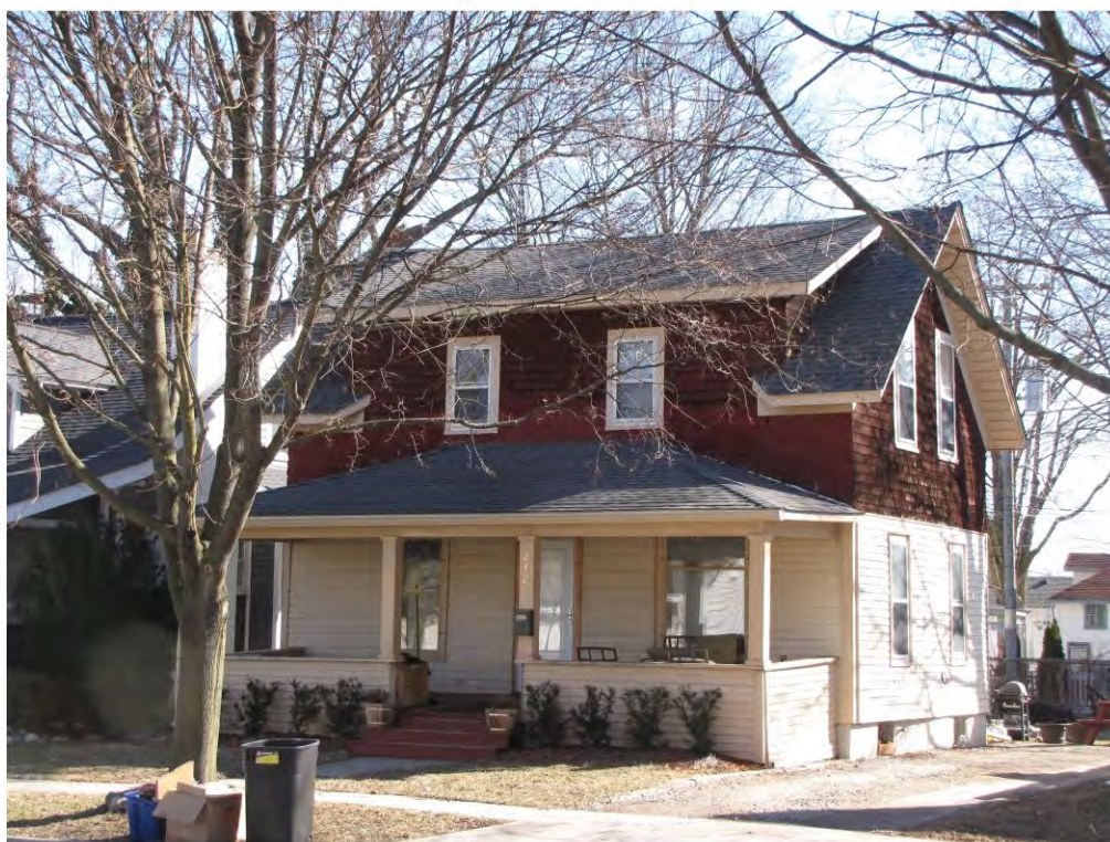
Wing North 212_Looking Northeast
