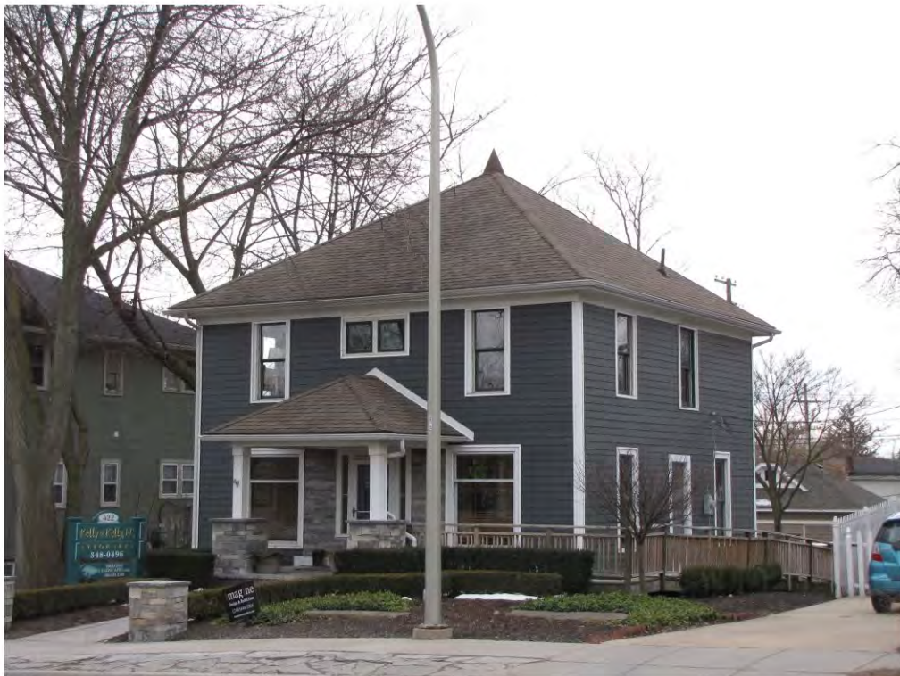
Main East 422_Looking Southeast
