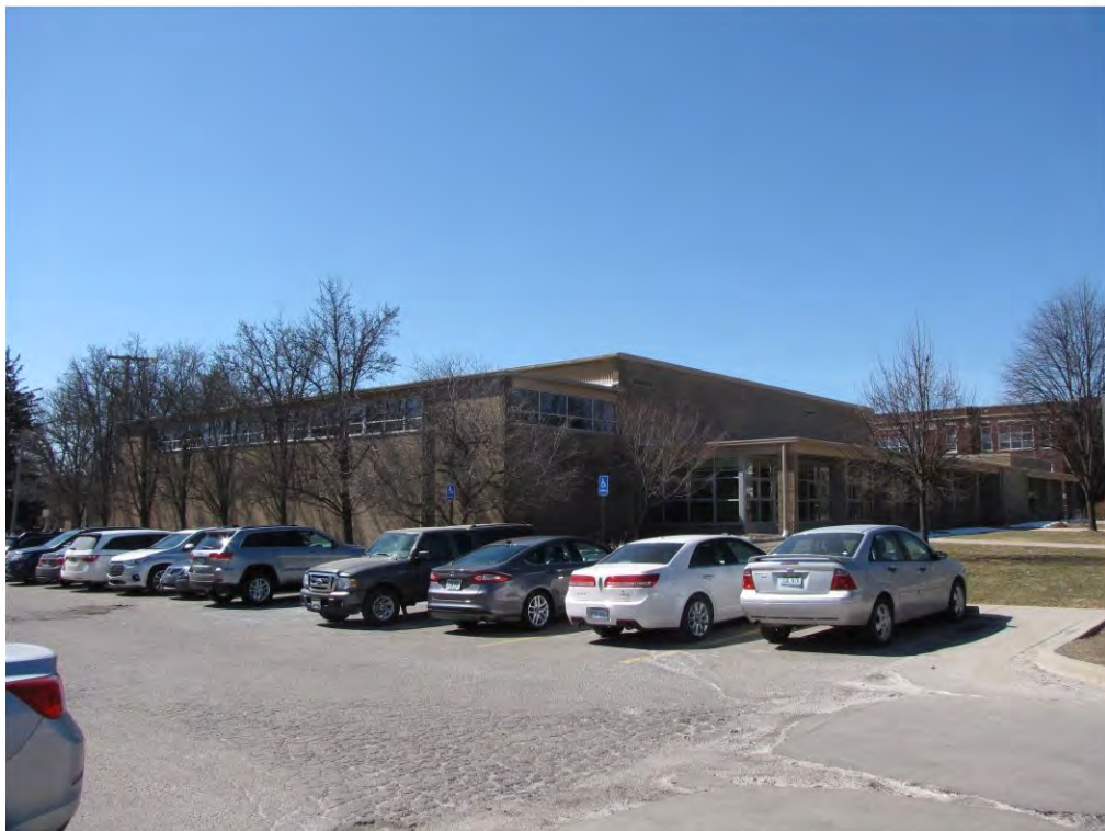
Main West 303_Looking Southwest
