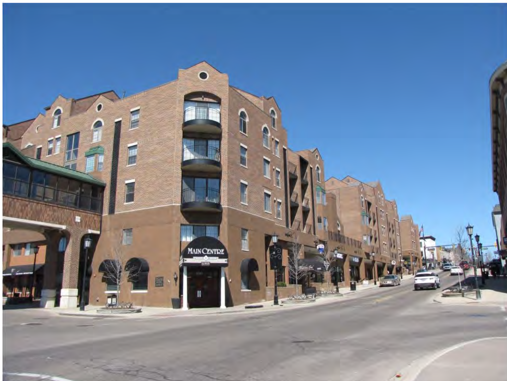
MainCentre 150_Looking Northwest
