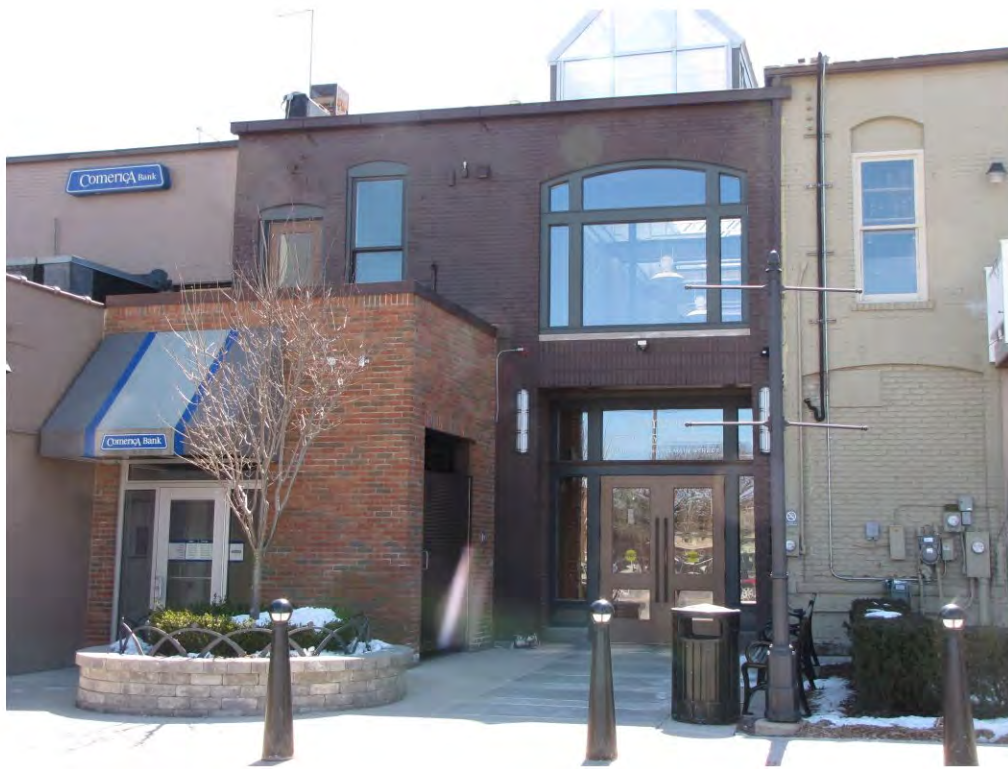
Main East 125_Looking South
