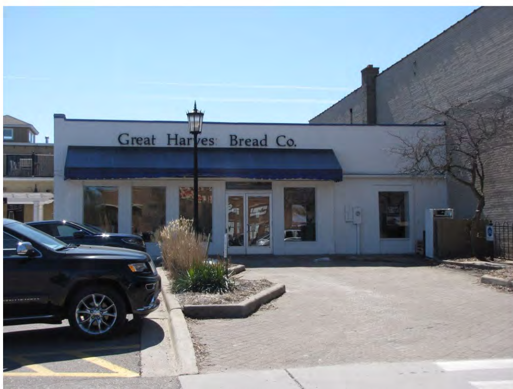
Main East 139_Looking South
