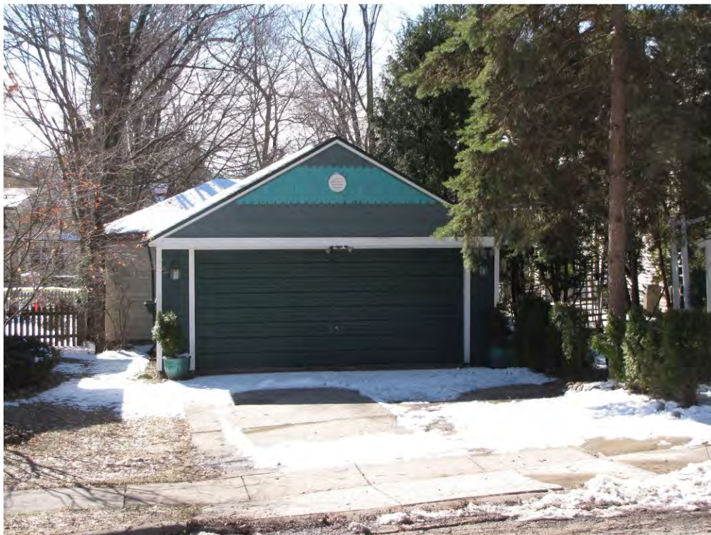
Rogers North 234, Garage_Looking South
