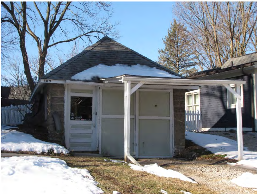
Randolph 509, Garage_Looking South
