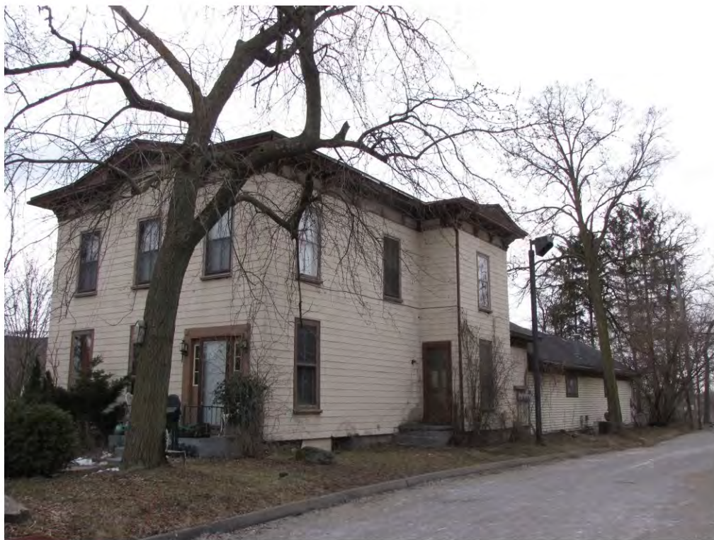
Main East 342_Looking Southeast
