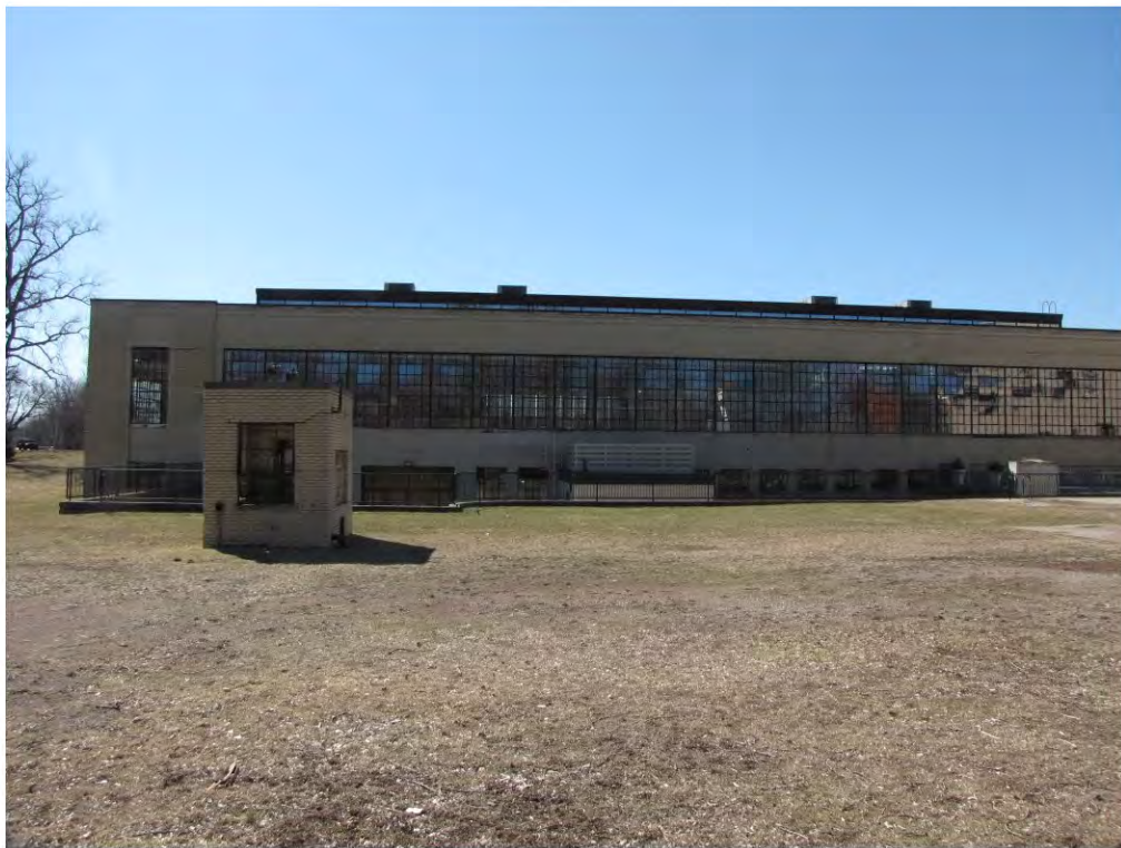
Main East 235_Looking South
