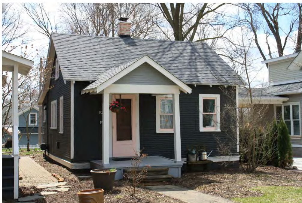
Main West 523_Looking Southwest
