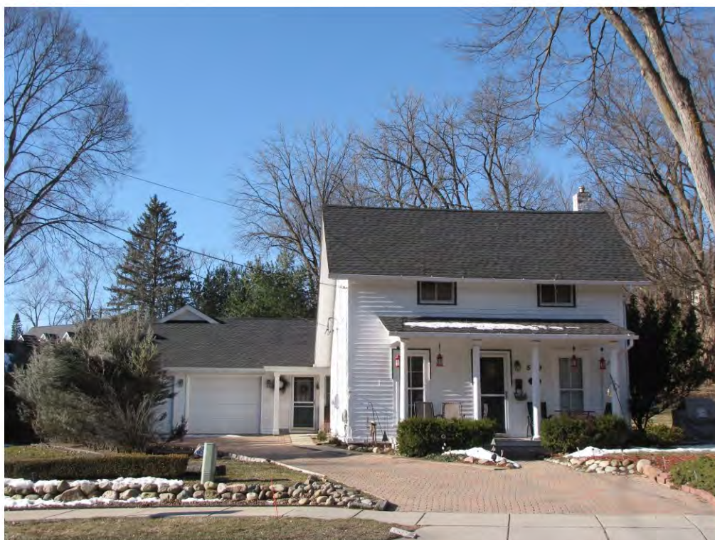
Randolph 529_ Looking South
