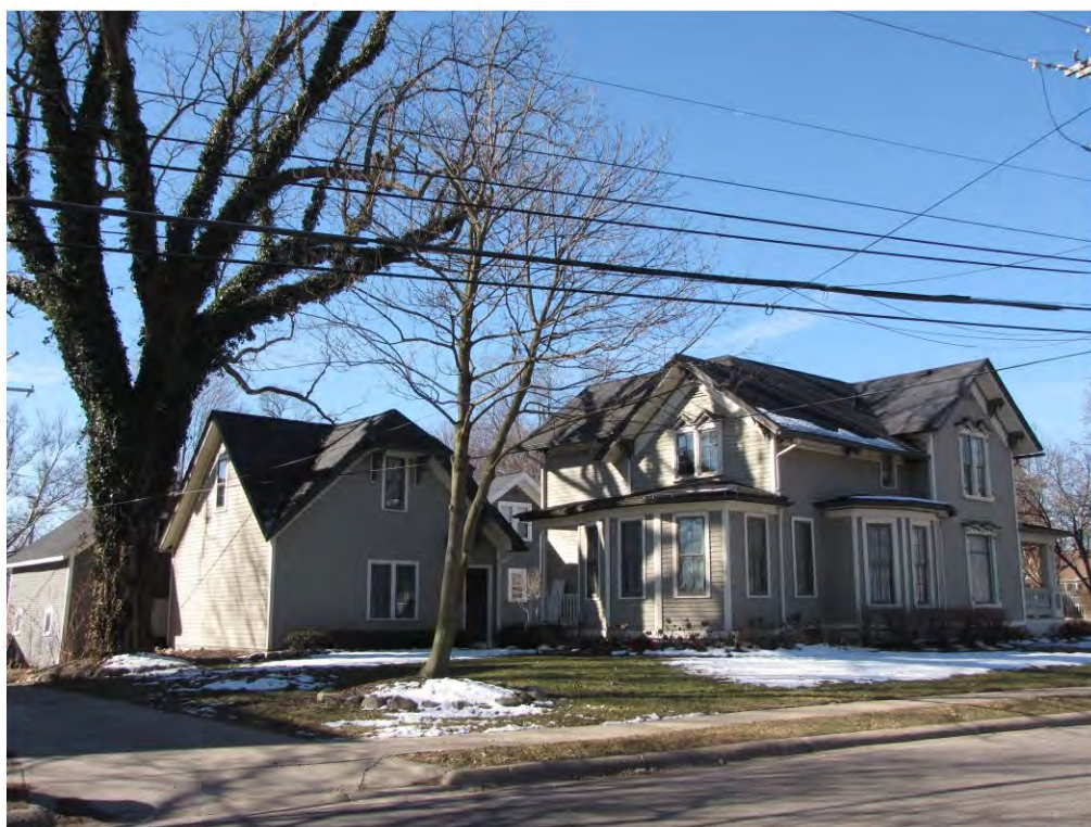
Wing North 220_Looking Northeast
