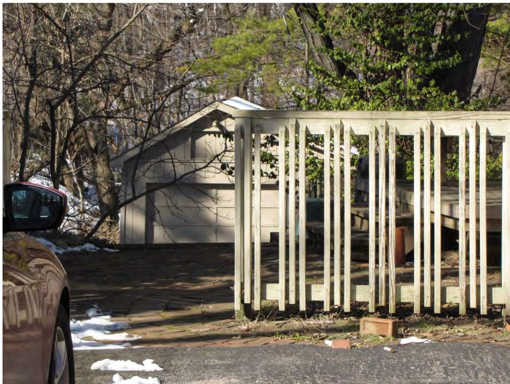
Randolph North 117, Garage_Looking West
