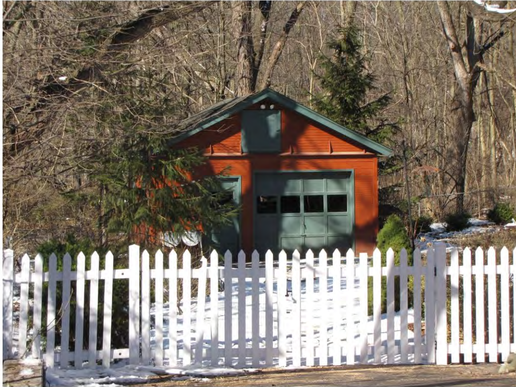
Rogers North 201, Garage_Looking West
