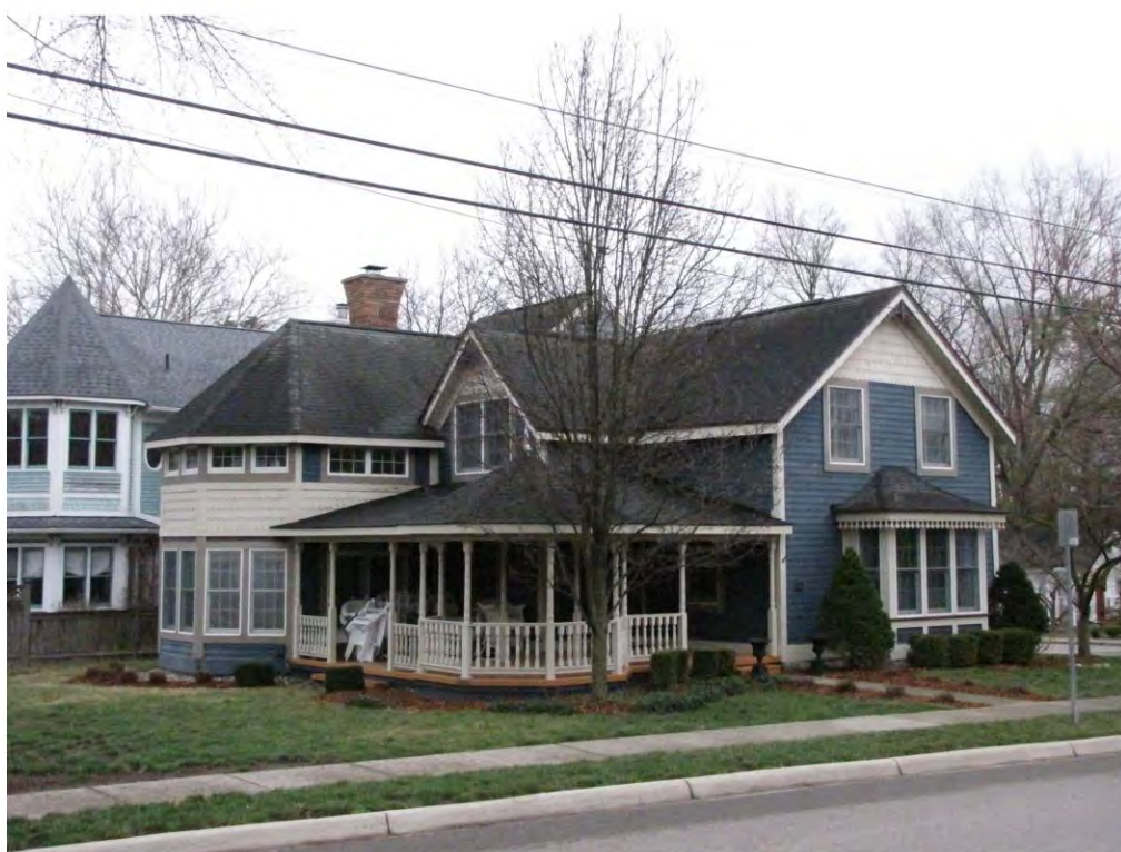
Rogers South 127_Looking Southeast
