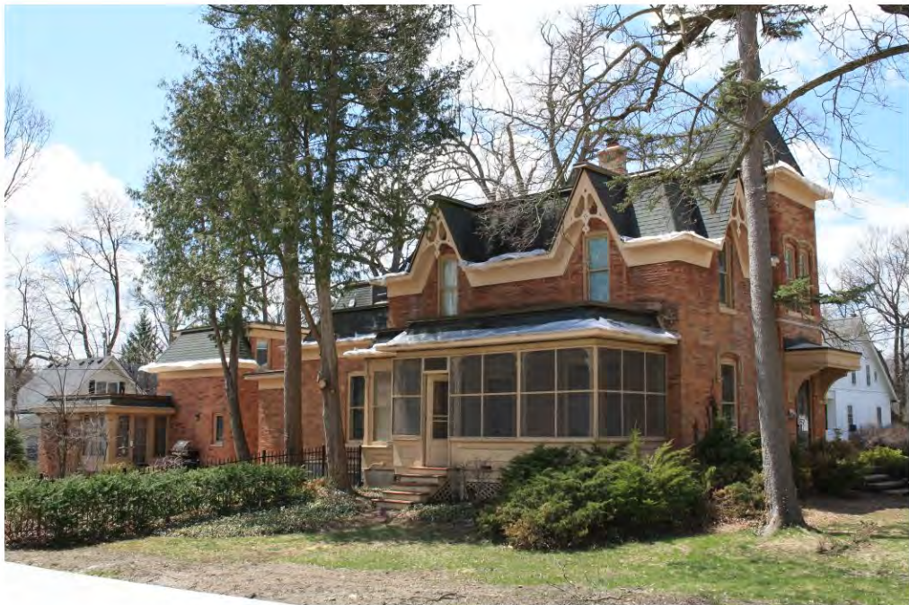
Main West 547_Looking Southwest
