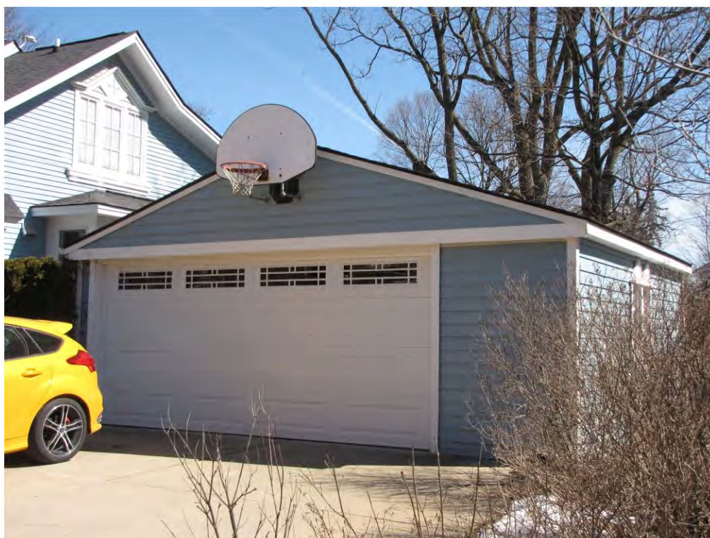
Dunlap West 417, Garage_Looking Northeast
