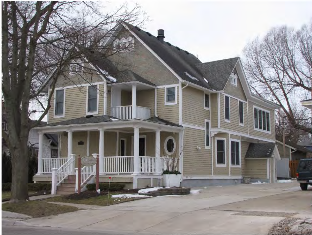
Wing North 117_Looking Southwest
