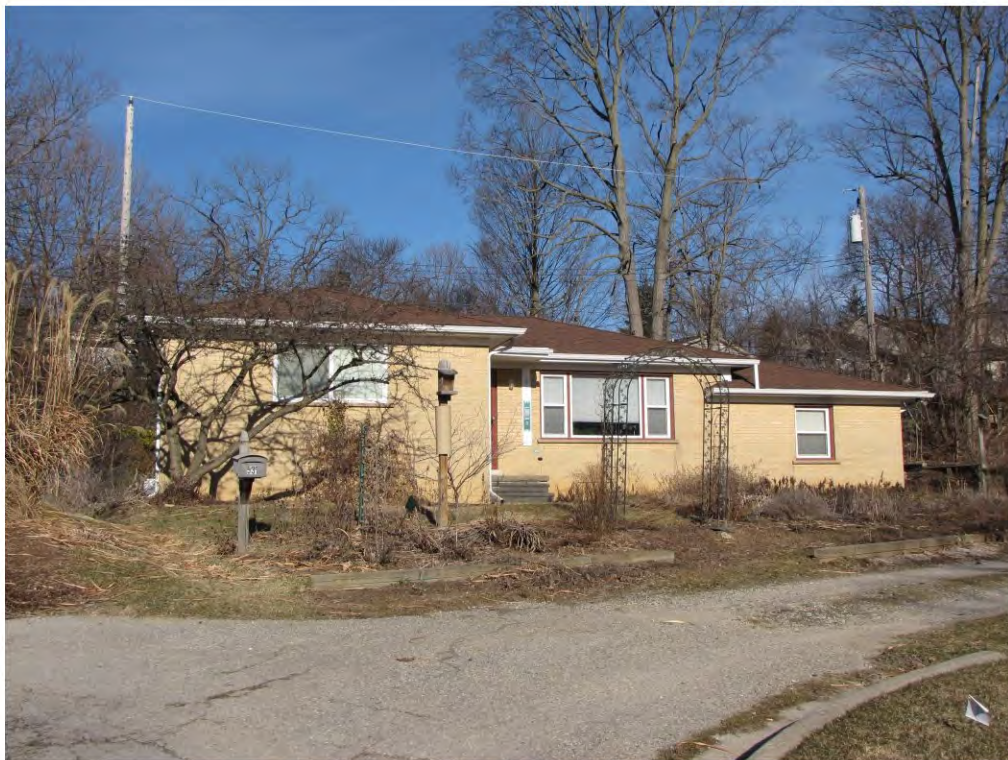
Linden Court 531_Looking Northwest
