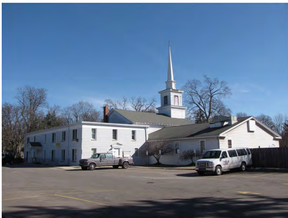
Wing North 217_Looking Northeast
