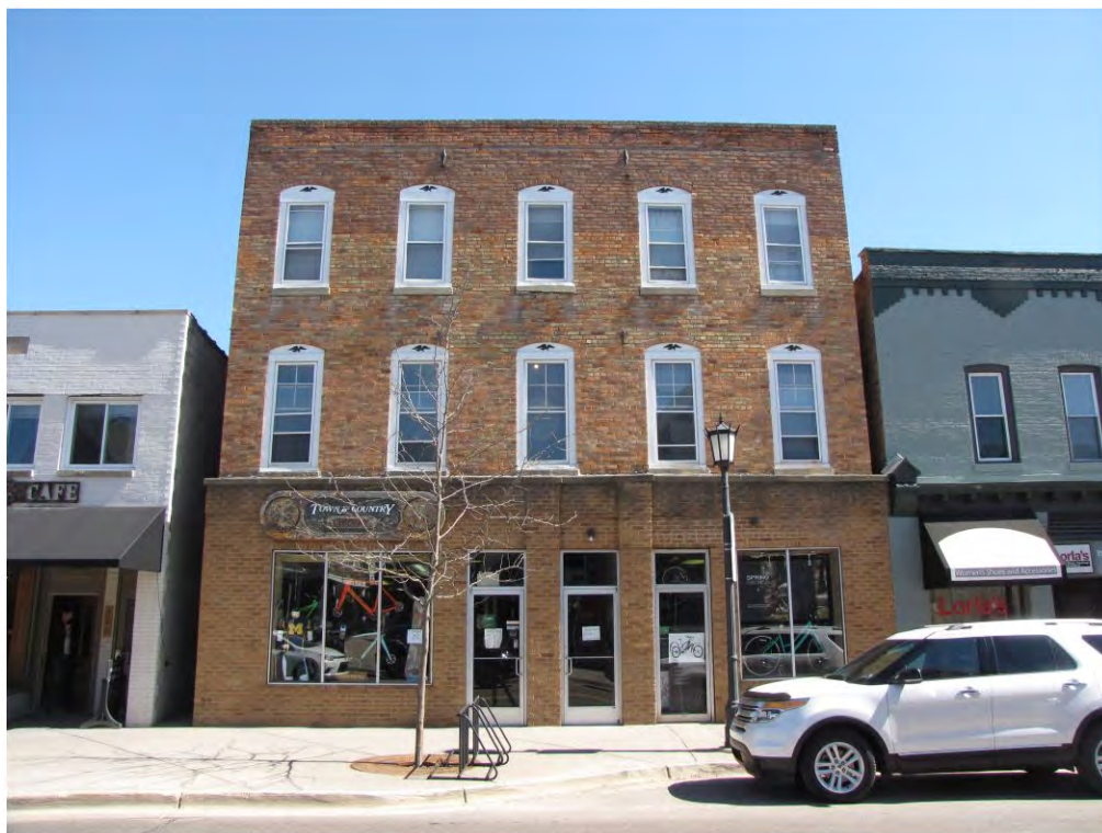
Center North 144-148_Looking East
