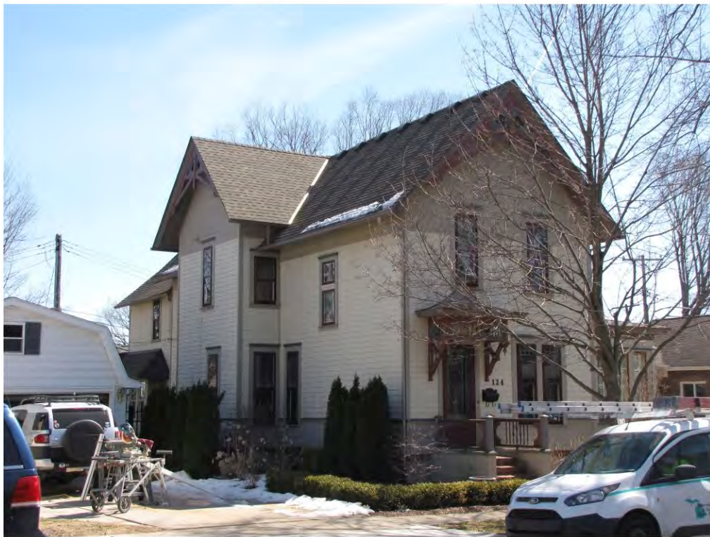
High 124_Looking Southeast
