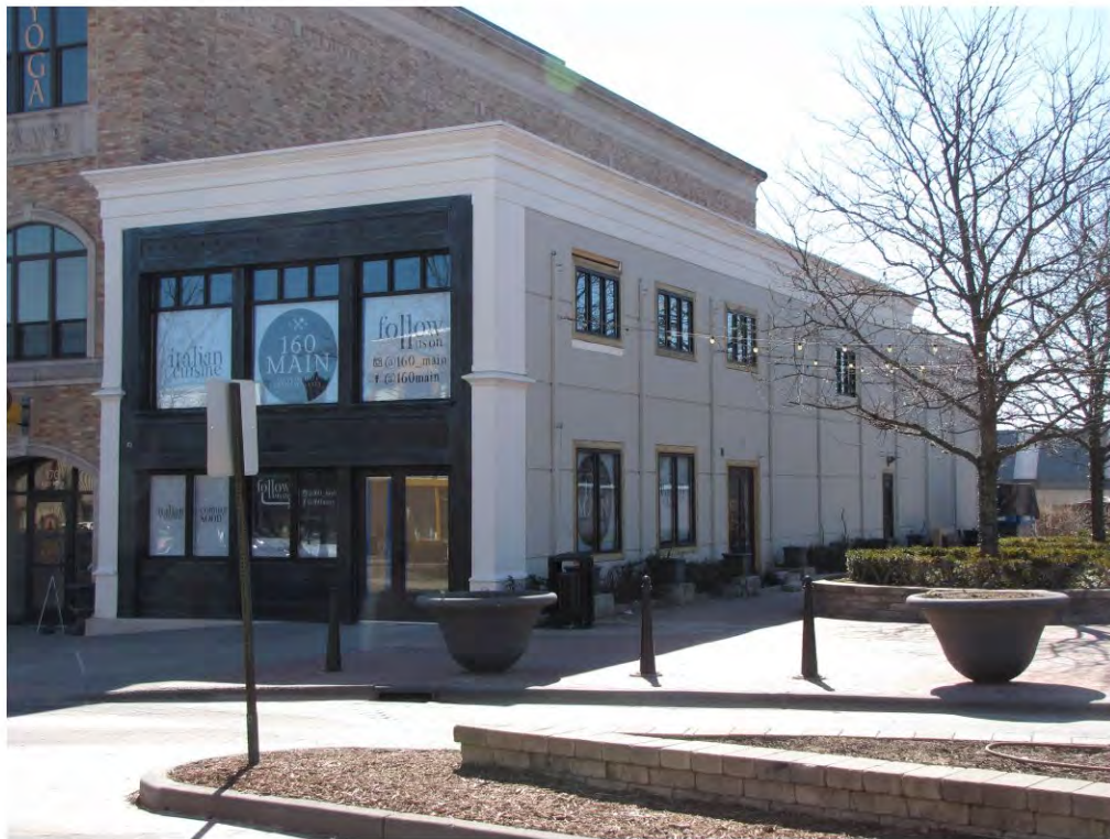
Main East 160_Looking Southeast
