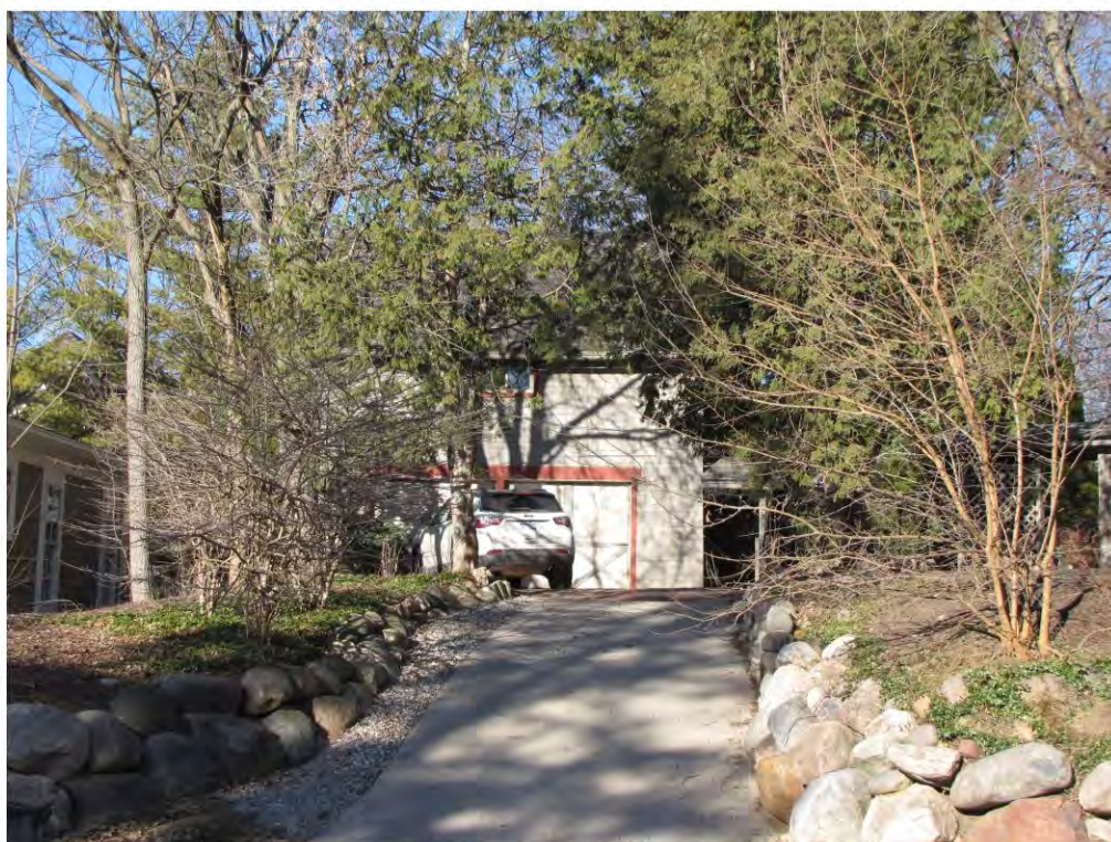
Randolph 503, Garage_Looking West
