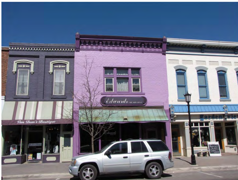
Main East 115_ Looking North
