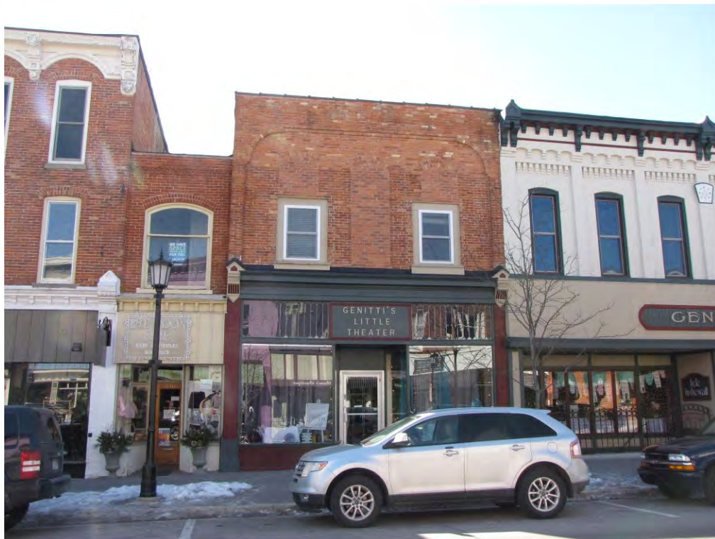
Main East 112_Looking South
