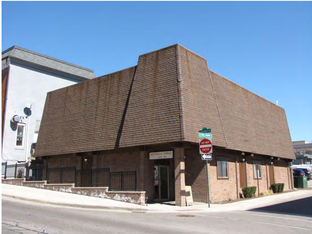
Center South 113_Looking Northeast
