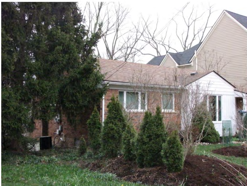
Rogers North 368_Looking Southeast
