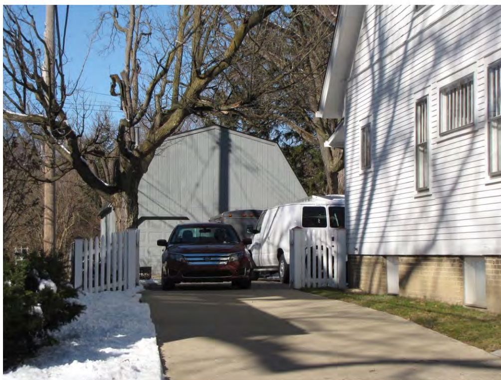
Rogers South 110, Garage_Looking West
