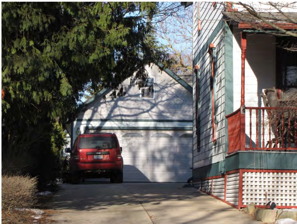
Rogers North 365, Garage_Looking West
