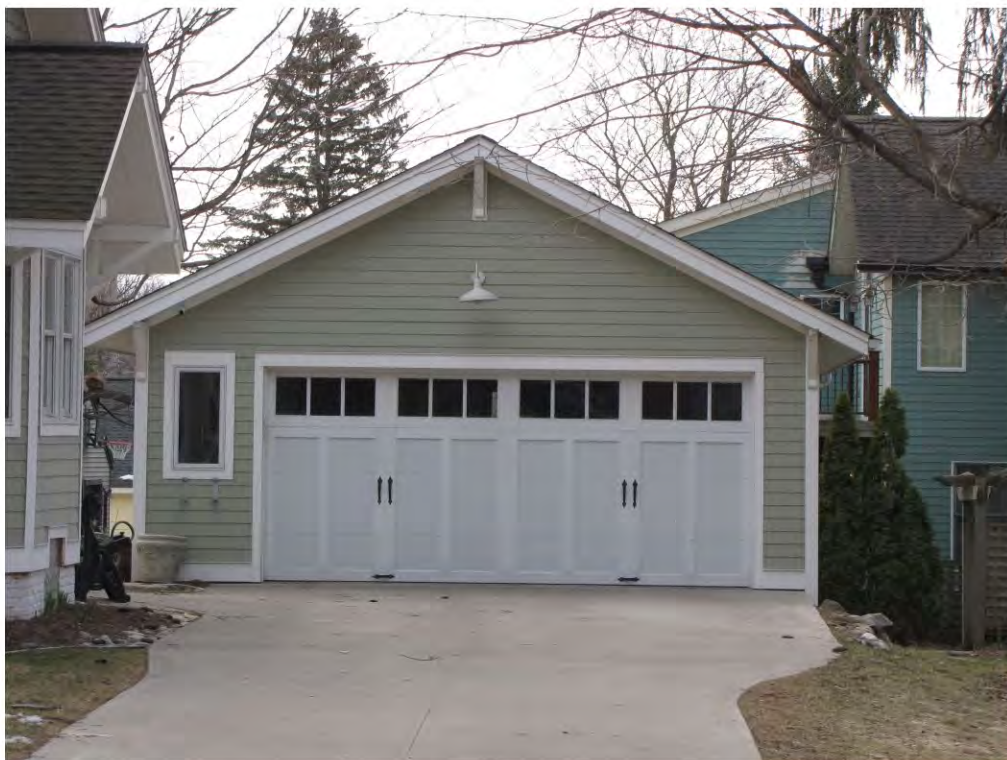
Cady West 487, Garage_Looking South
