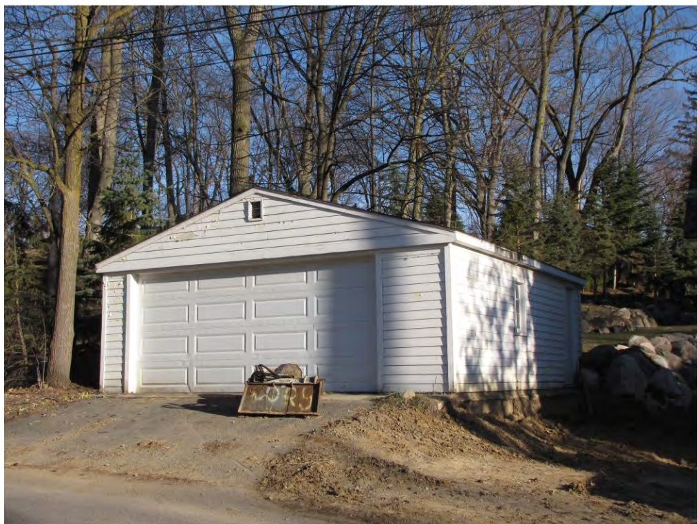
Rogers North 333, Garage_Looking Northwest
