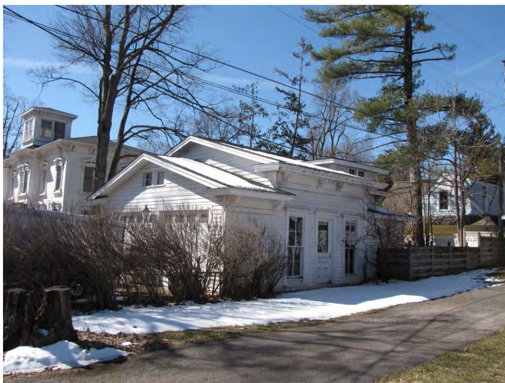
Dunlap West 404, Garage_Looking Southwest
