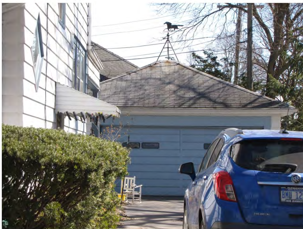
West 114, Garage_Looking East
