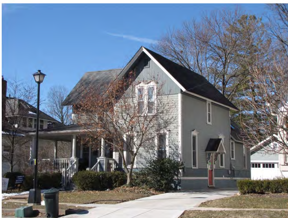
High 229_Looking Southwest
