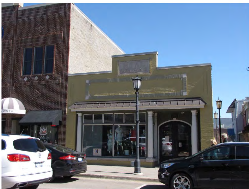
Center North 120_Looking East
