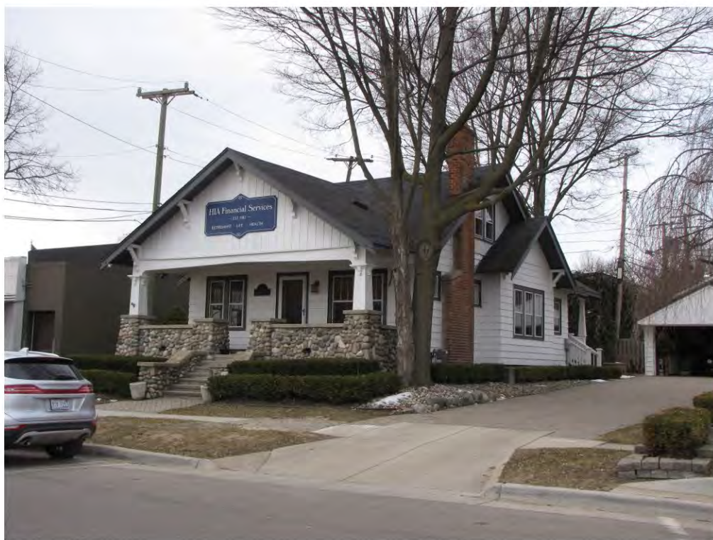
Wing North 111_Looking Southwest
