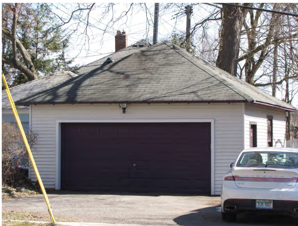
Main West 312, Garage_ Looking East
