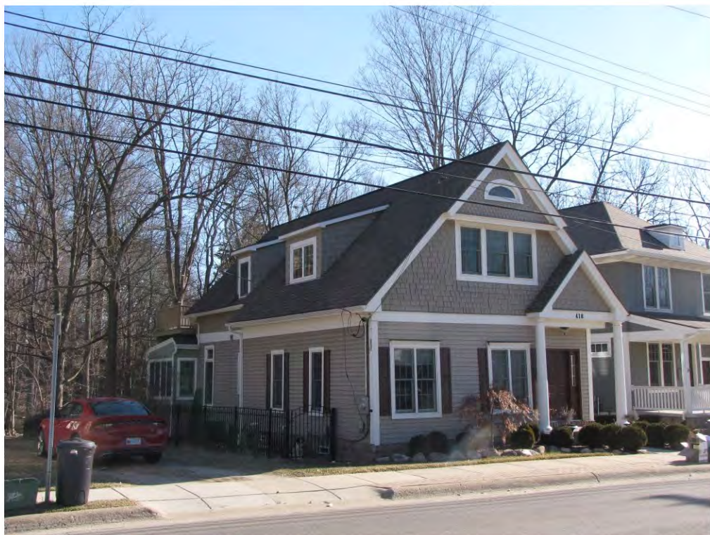
Randolph 418_Looking Northeast
