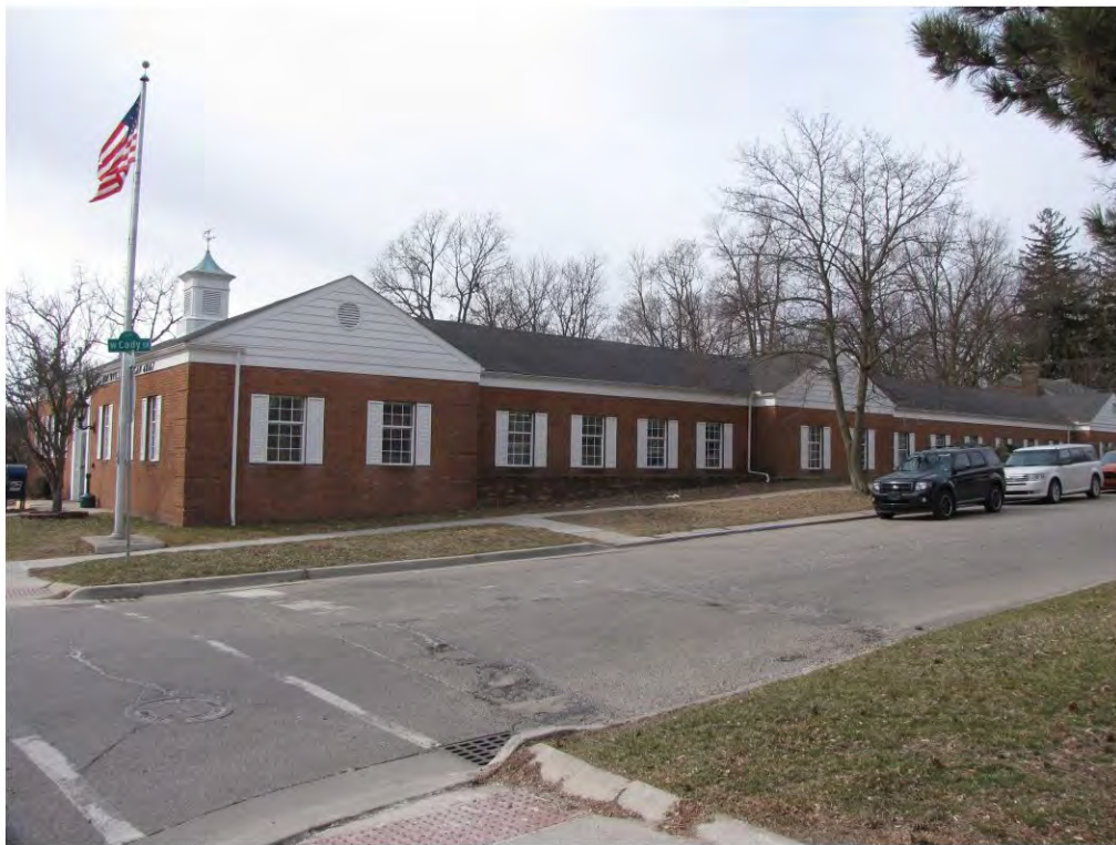
Wing South 200_Looking Southwest
