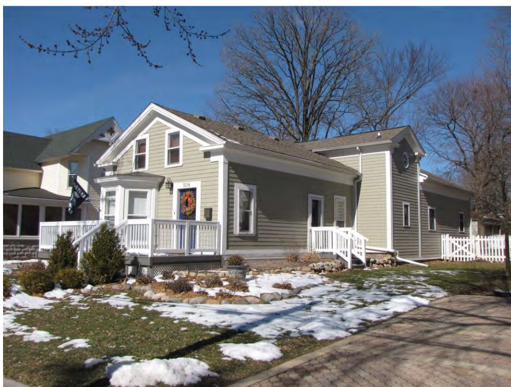
Main West 508_Looking Northwest
