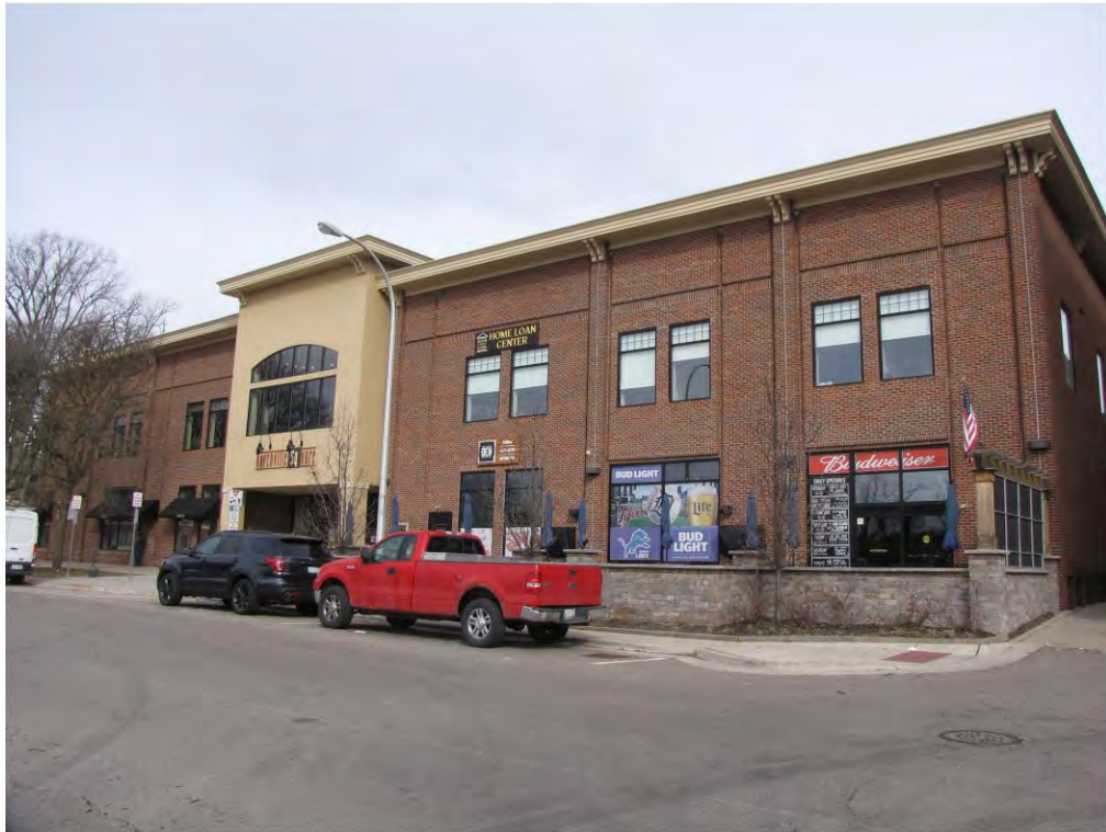
Main West 133_Looking Northwest
