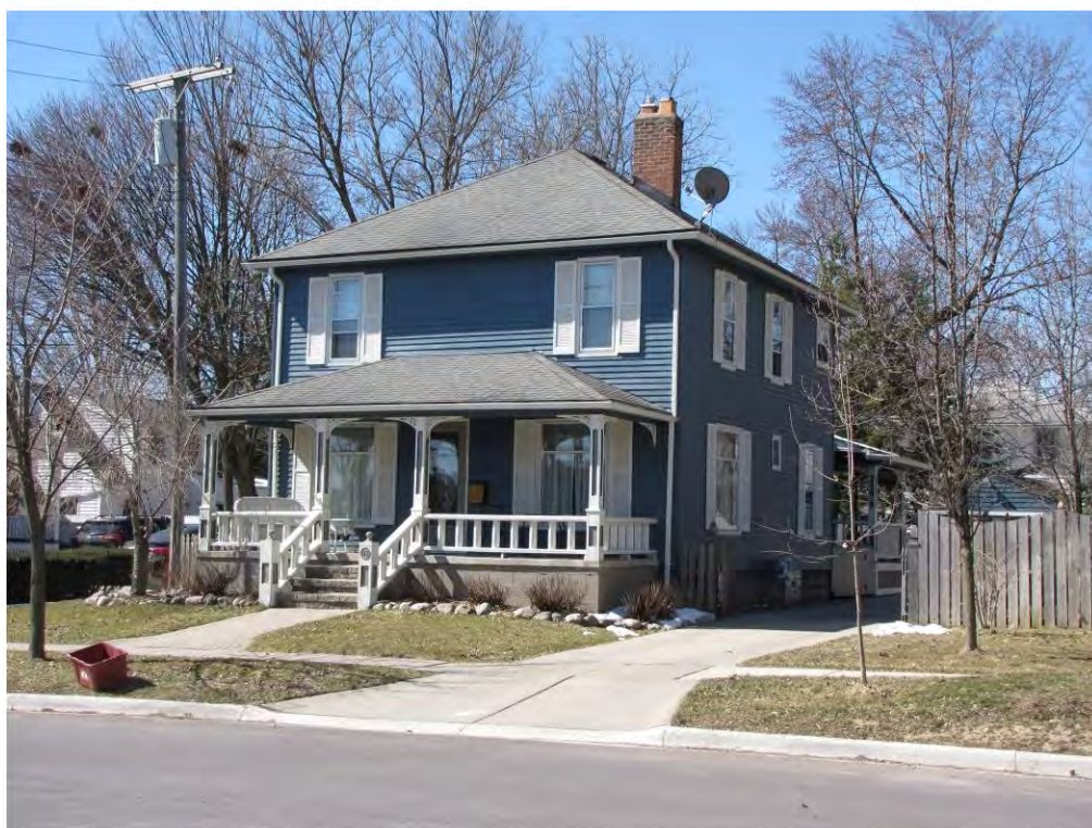
High 113_Looking Southwest
