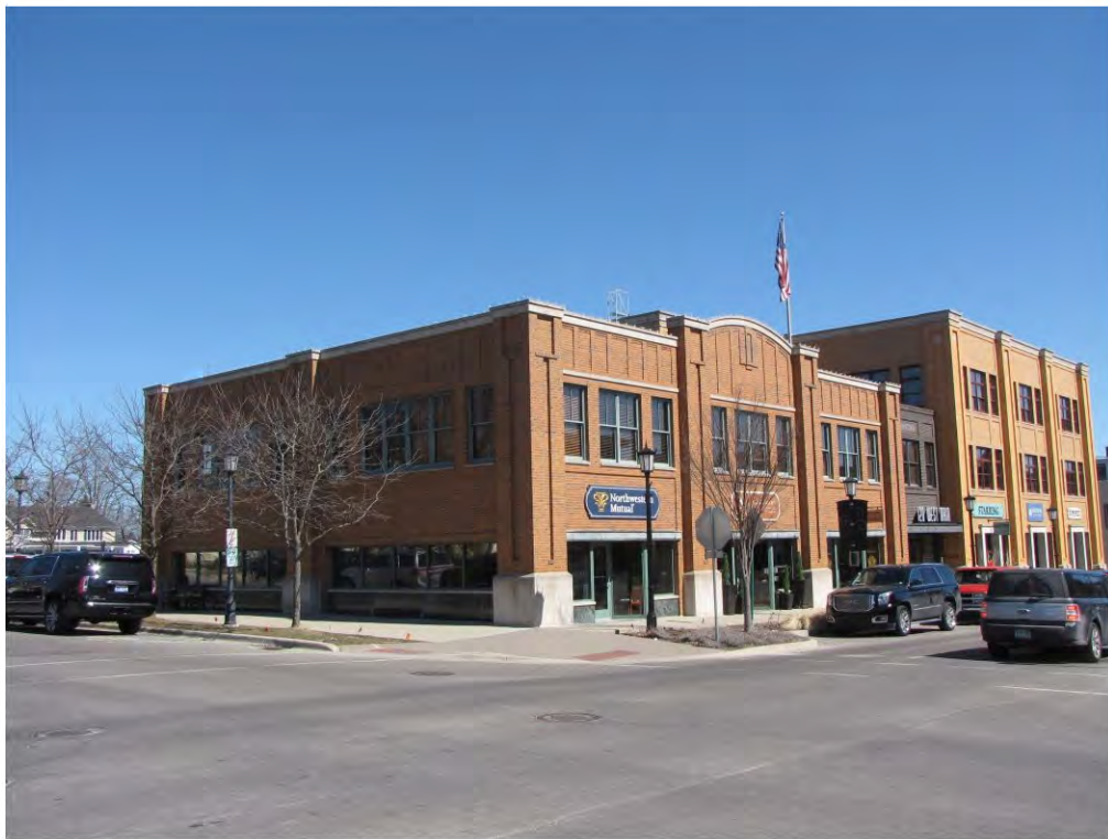
Main West 114-126_Looking Northeast
