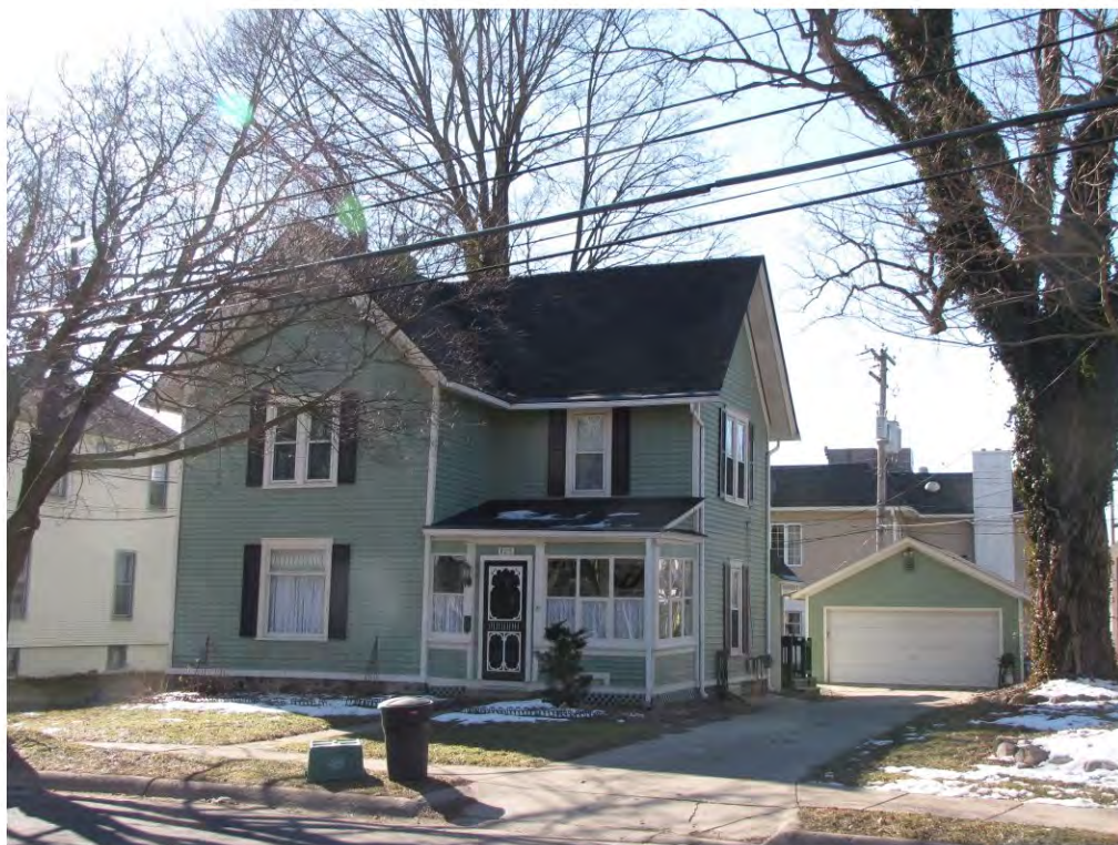
Randolph 125, Garage_Looking South
