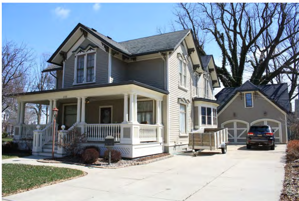
Wing North 220_Looking Southwest
