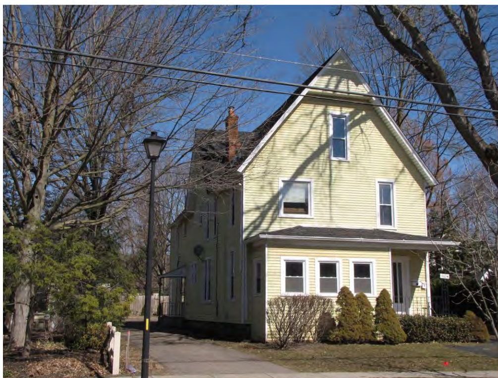
Main West 410_Looking Northeast
