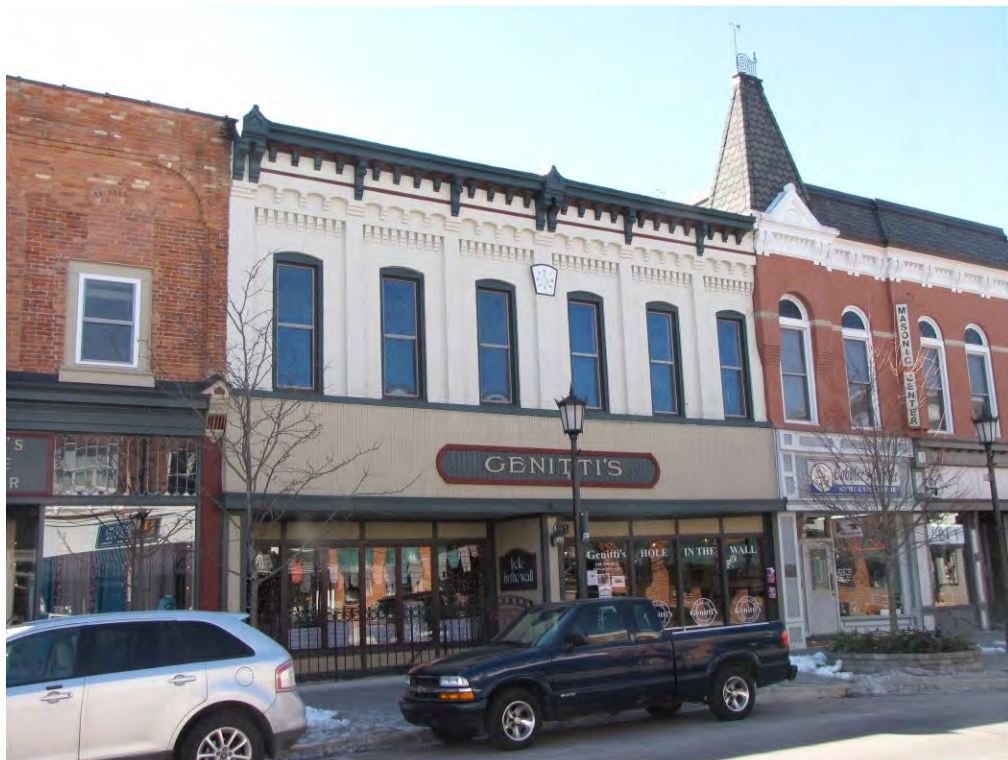
Main East 108-110_Looking Southeast
