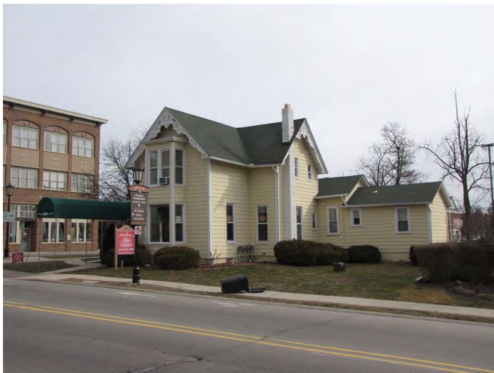
Center South 201 and Cady East 100_Looking Northeast
