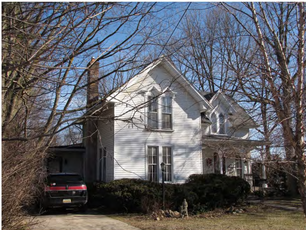
Randolph 132_Looking Northeast
