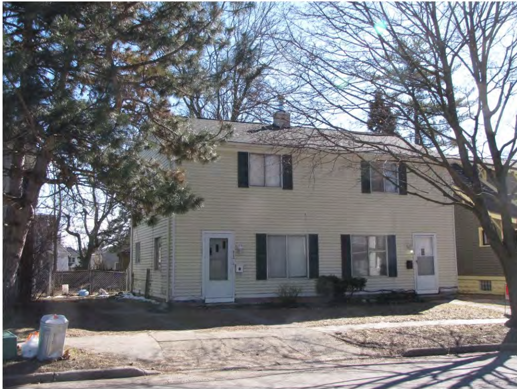
Linden 222-224_ Looking Southeast
