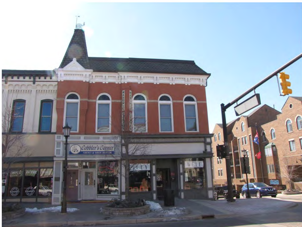
Main East 102-106 and Center South 113_Looking South
