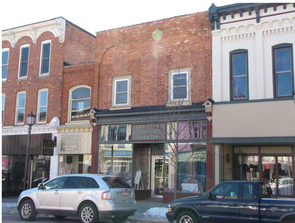
Main East 112_Looking Southeast
