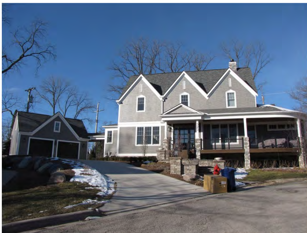
Linden Court 525_Looking Southwest
