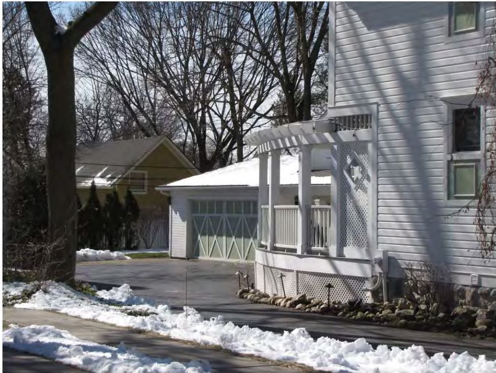
Dunlap West 537, Garage_Looking Southwest
