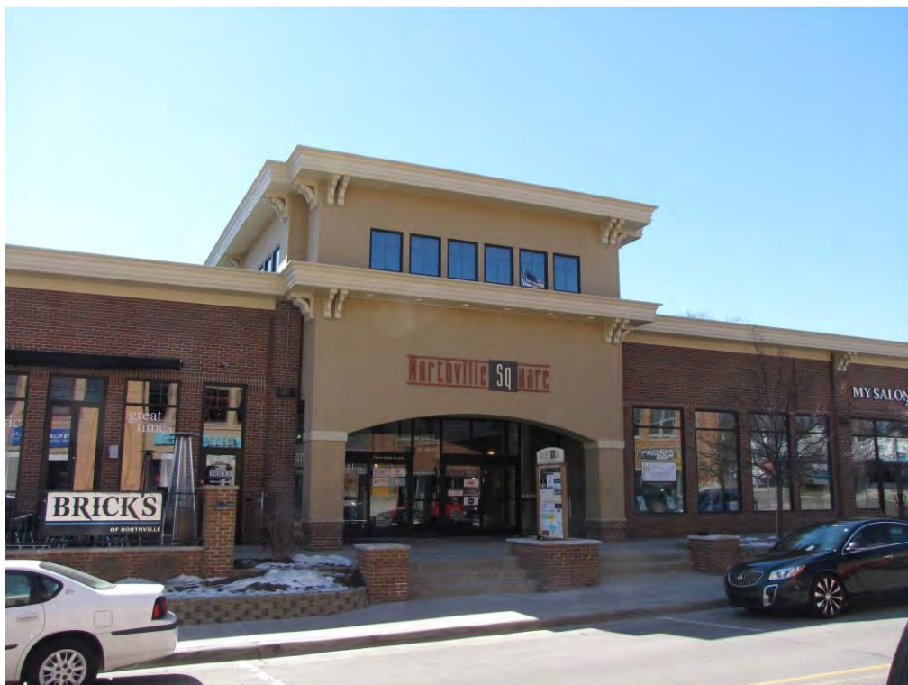
Main West 133_Looking South
