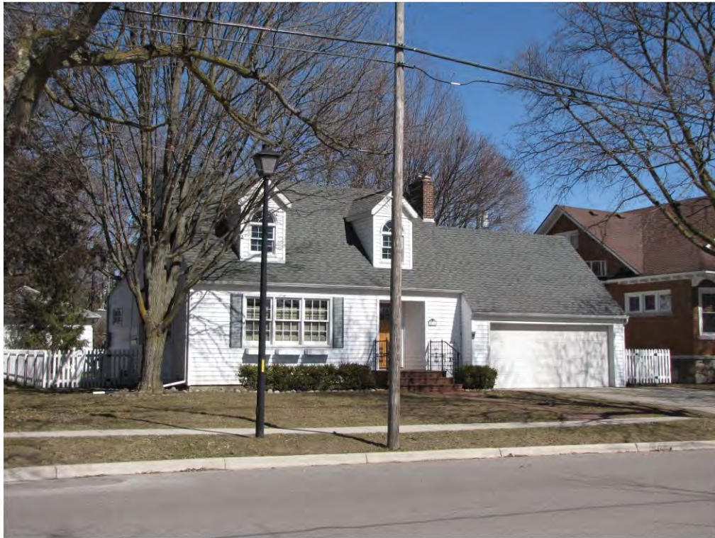
Main West 306_Looking Northeast
