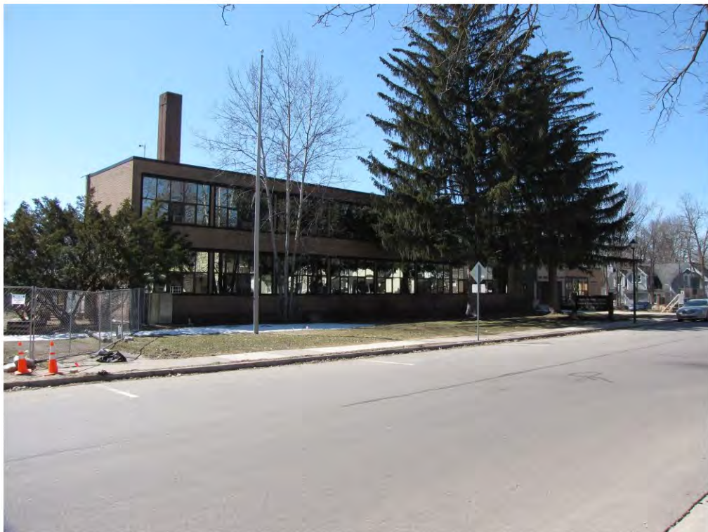
Main West 501_Looking Southwest
