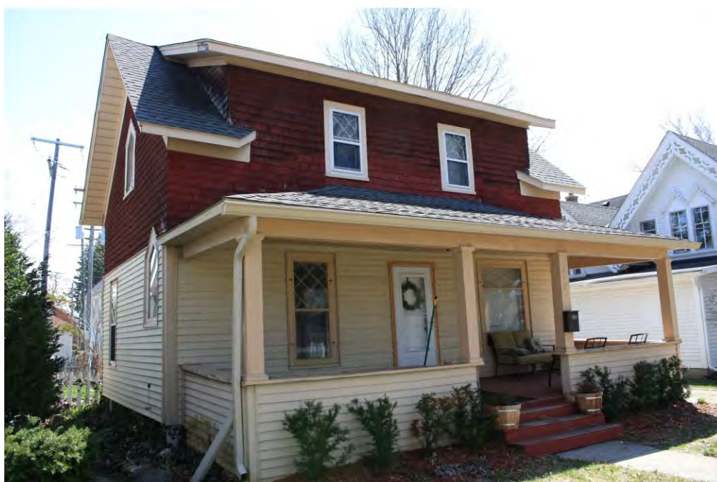
Wing North 212_Looking Southeast
