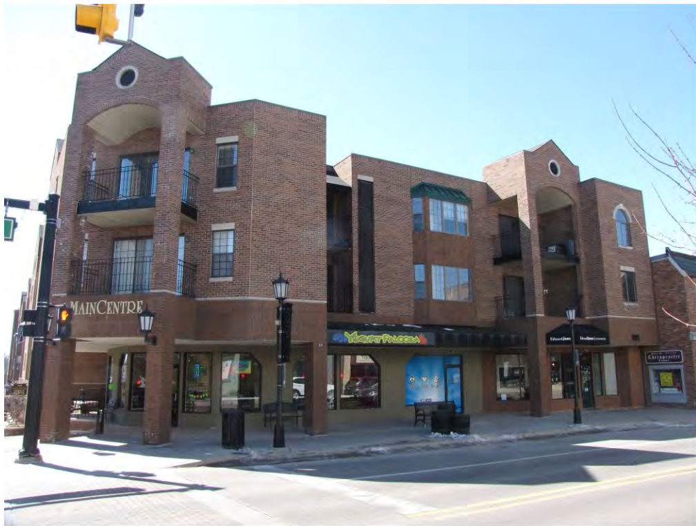
MainCentre 150_Looking Southwest
