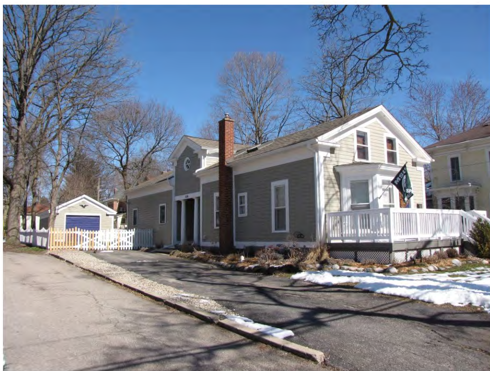
Main West 508_Looking Northeast
