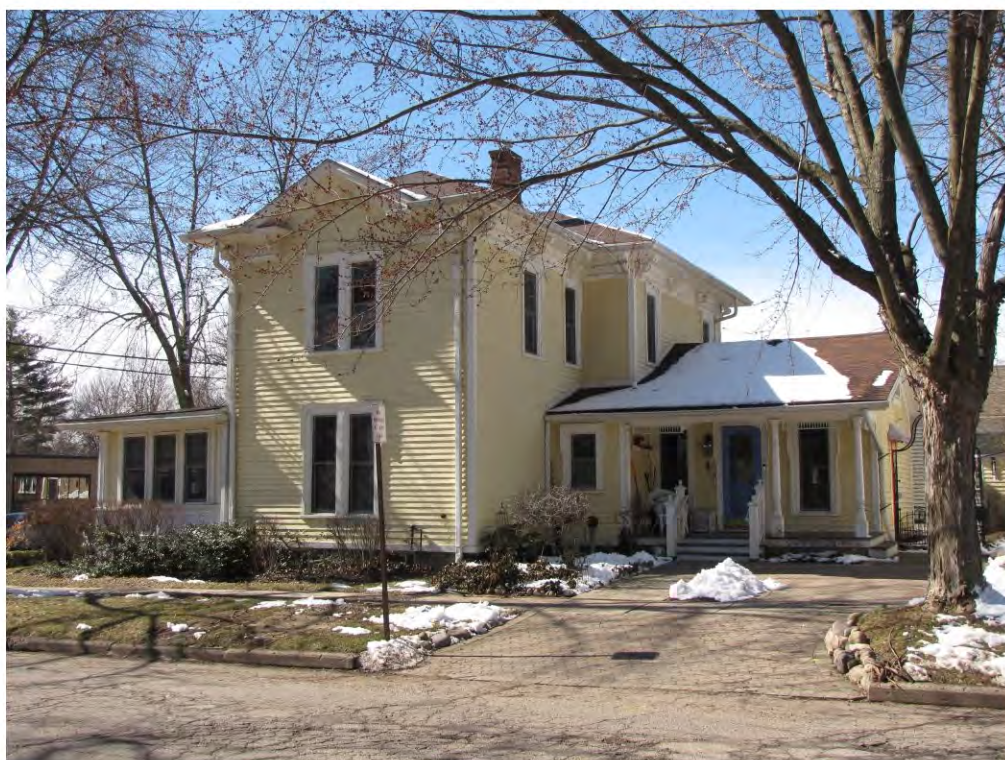
Main West 502_Looking Northeast
