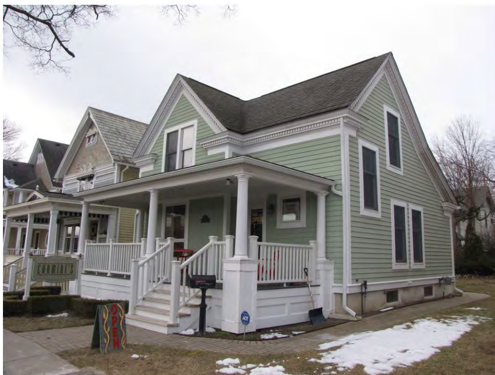
Wing North 125_ Looking Southwest
