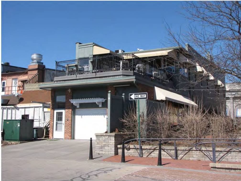
Main East 126-134_Looking South
