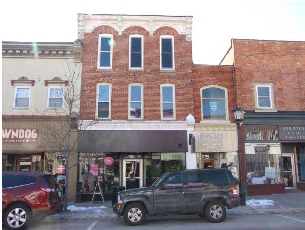
Main East 118_Looking South
