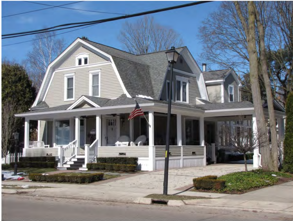
Main West 542_Looking Northwest
