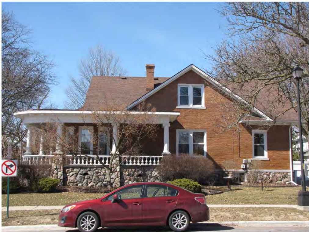
Main West 302_Looking West
