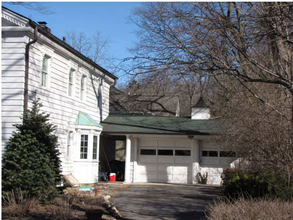
Randolph 204, Garage_Looking North
