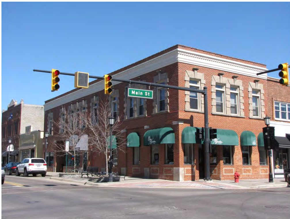
Main East 101 and Center North 108-110_Looking Northeast
