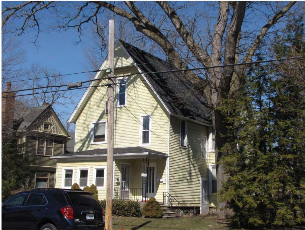
Main West 410_Looking Northwest
