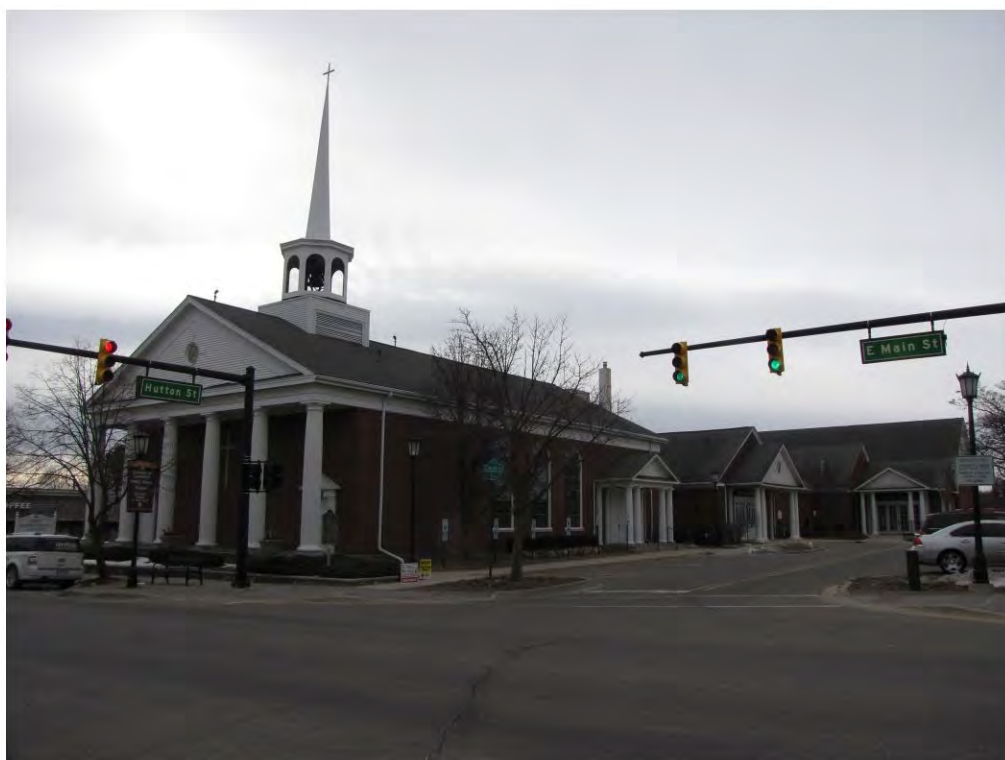
Main East 200_Looking Southeast
