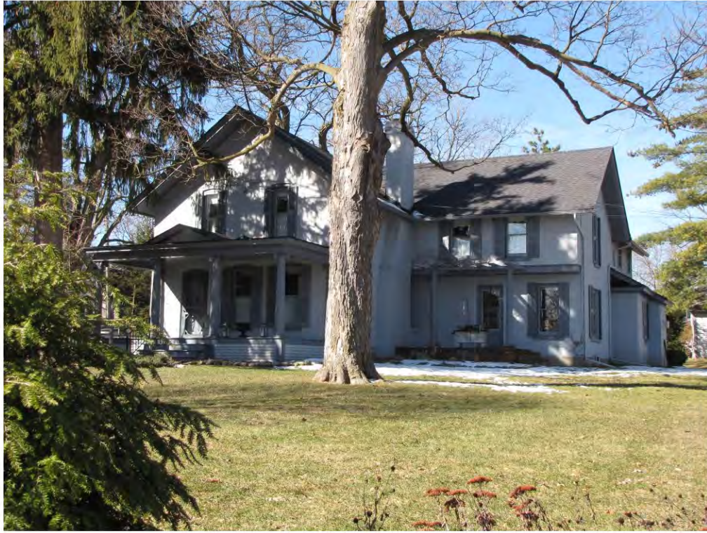
High 239_Looking Southwest
