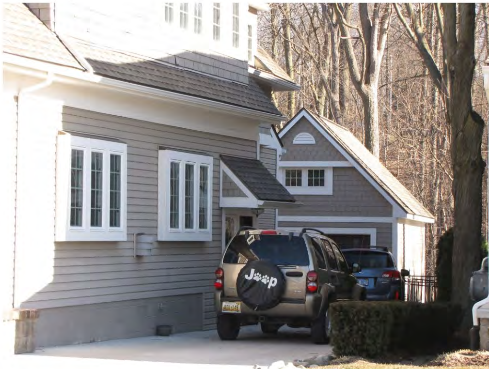
Randolph 418, Garage_Looking North
