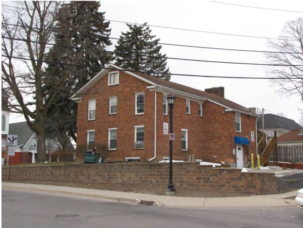
Dunlap West 100_ Looking Southwest
