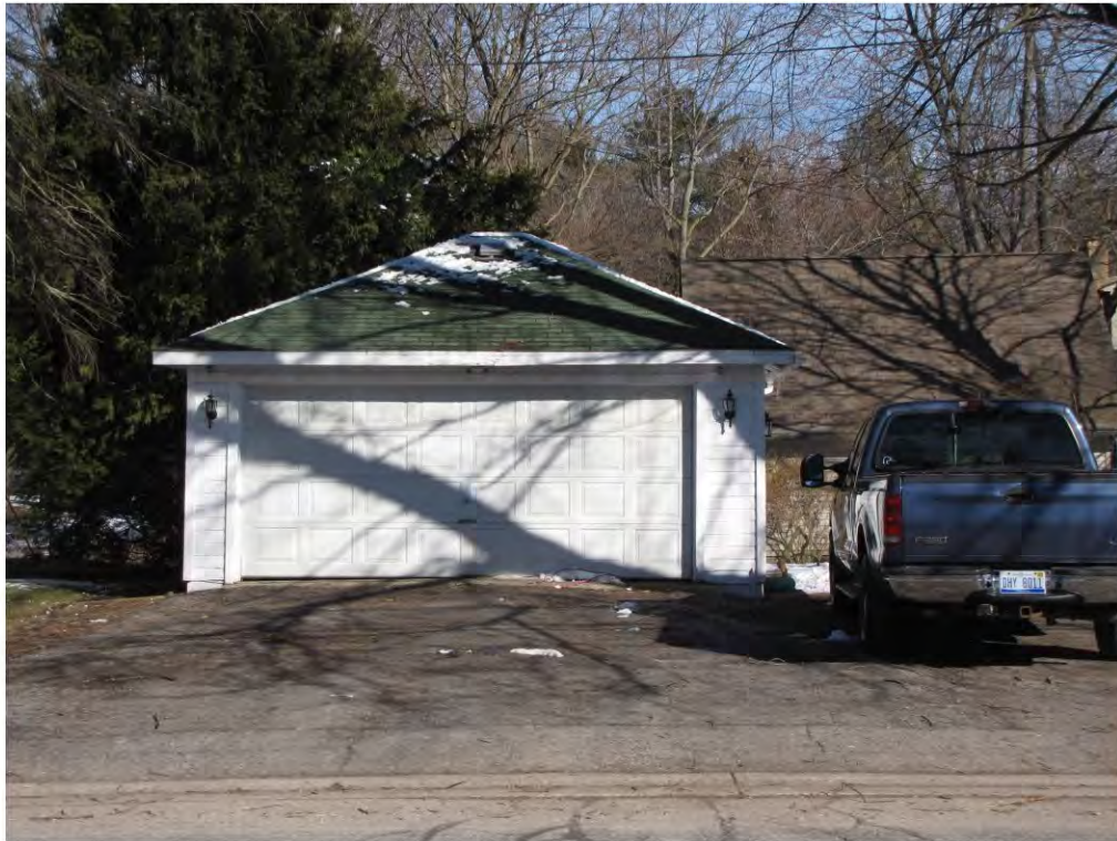
Rogers North 101, Garage_Looking North
