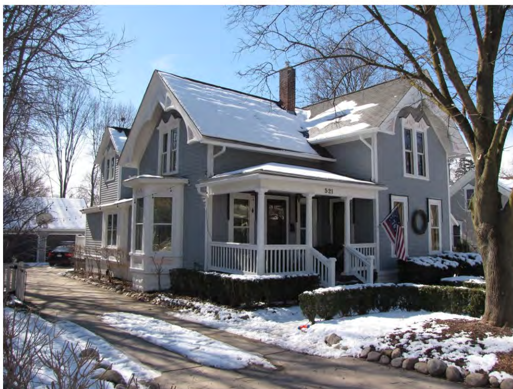
Main West 521_Looking Southwest
