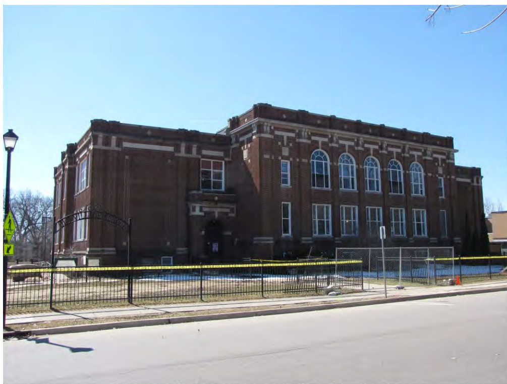
Main West 411_Looking South
