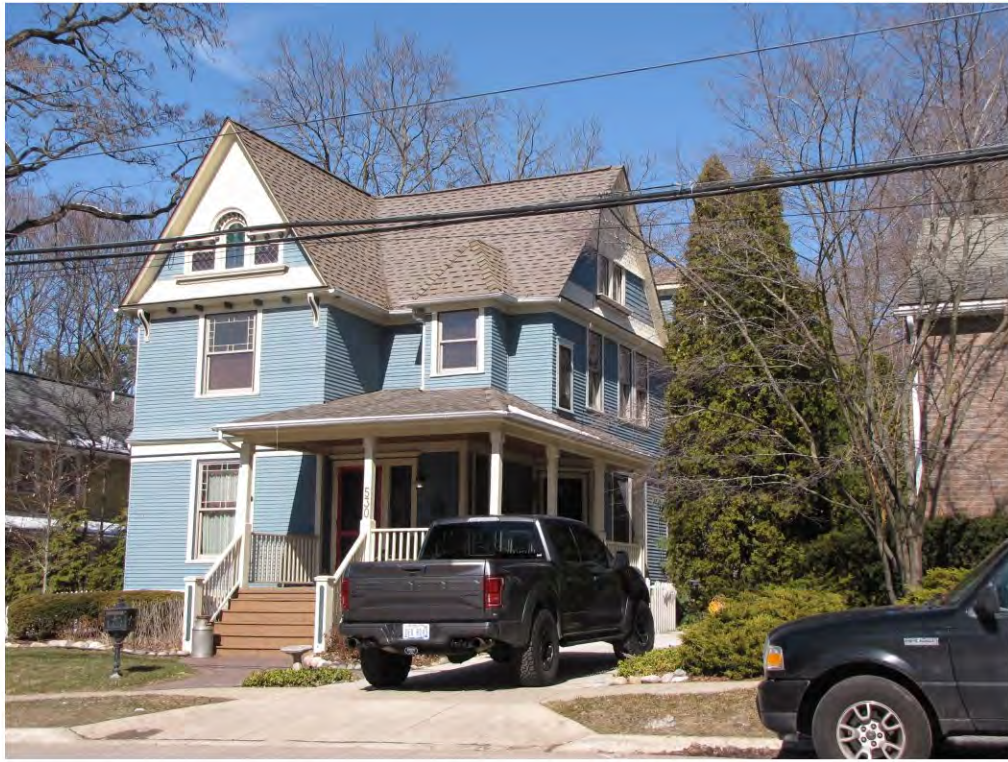
Main West 530_ Looking Northwest
