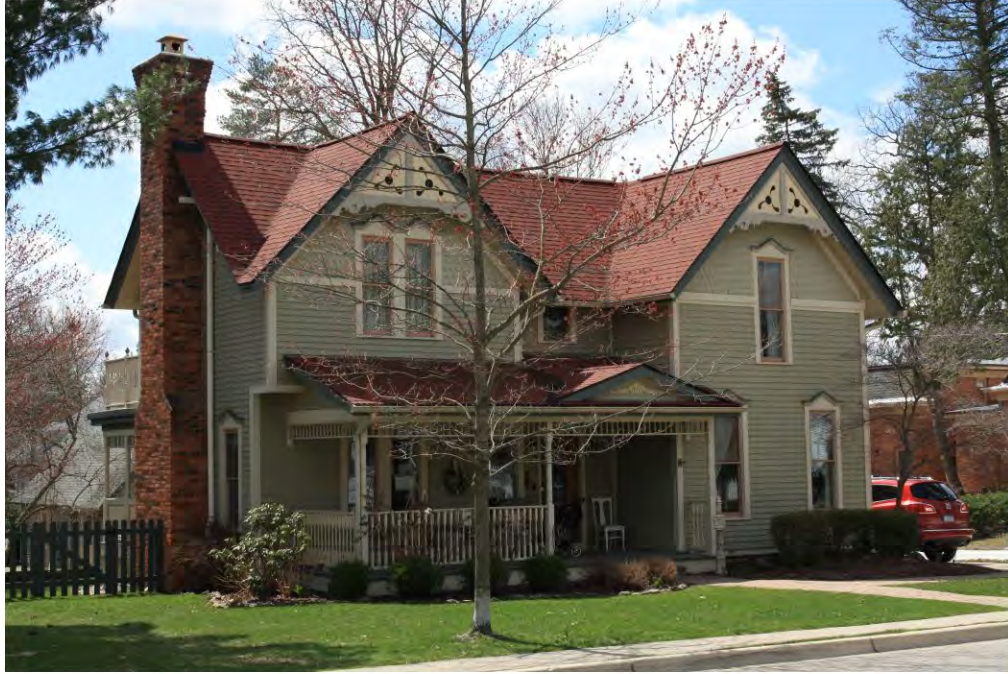
Main West 537_Looking Southwest
