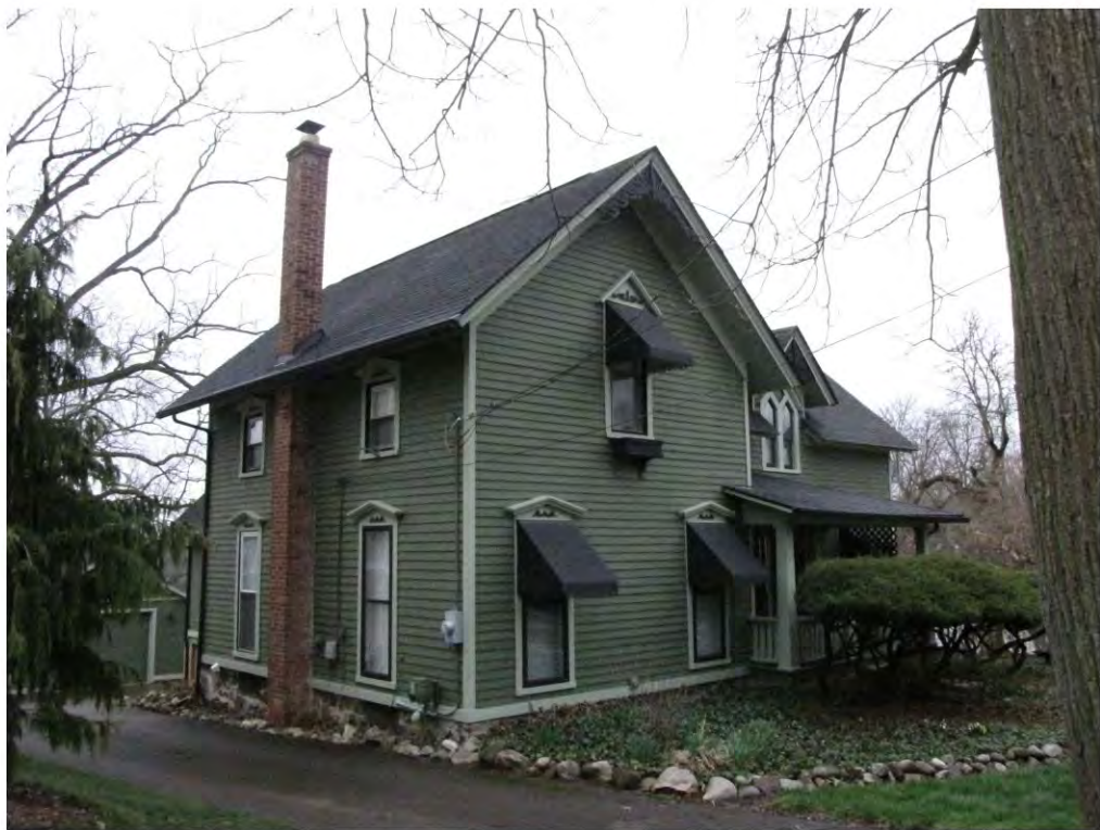
Rogers North 322_Looking Southeast
