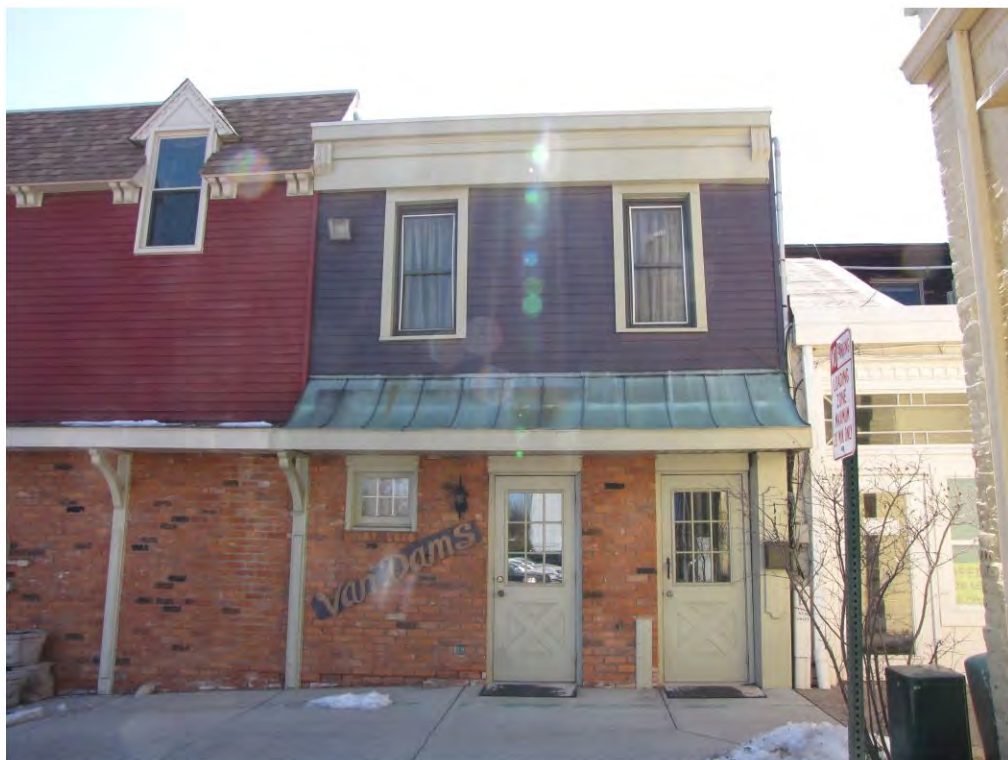
Main East 111_Looking South
