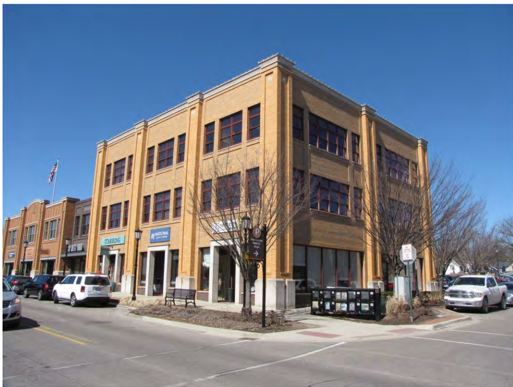
Main West 114-126_Looking Northwest
