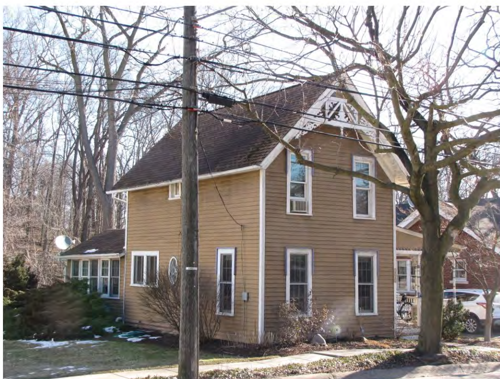
Randolph 442_Looking Northeast
