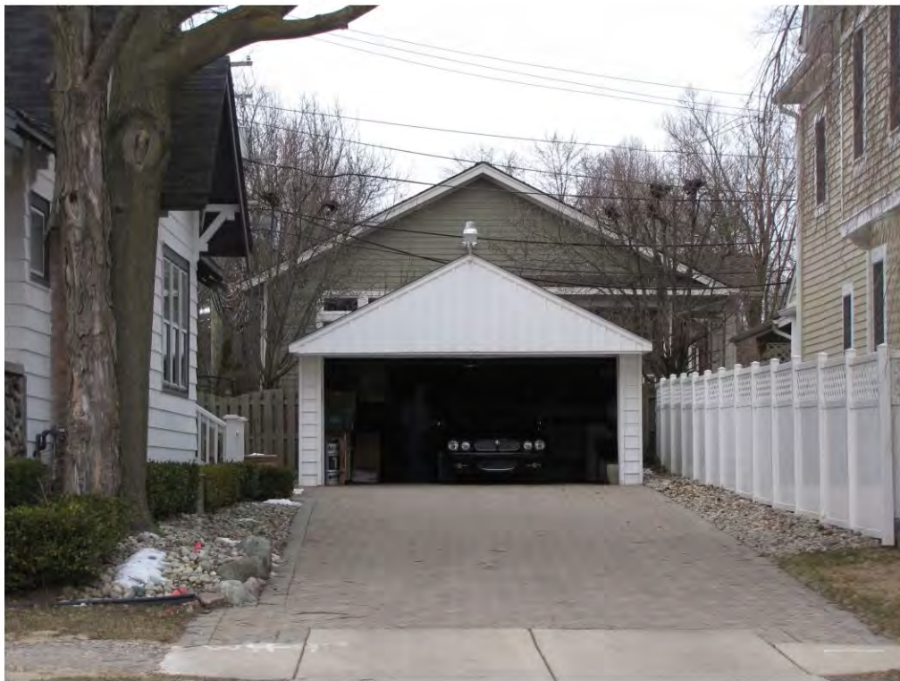
Wing North 111, Garage_Looking West
