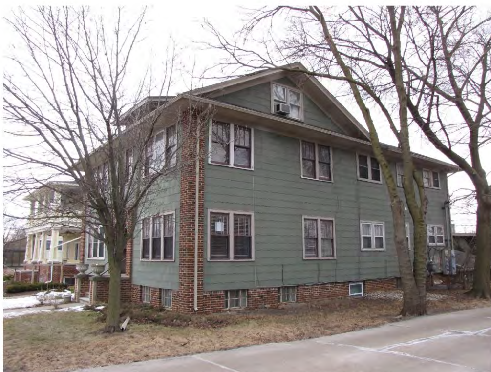
Main East 430_Looking Southeast
