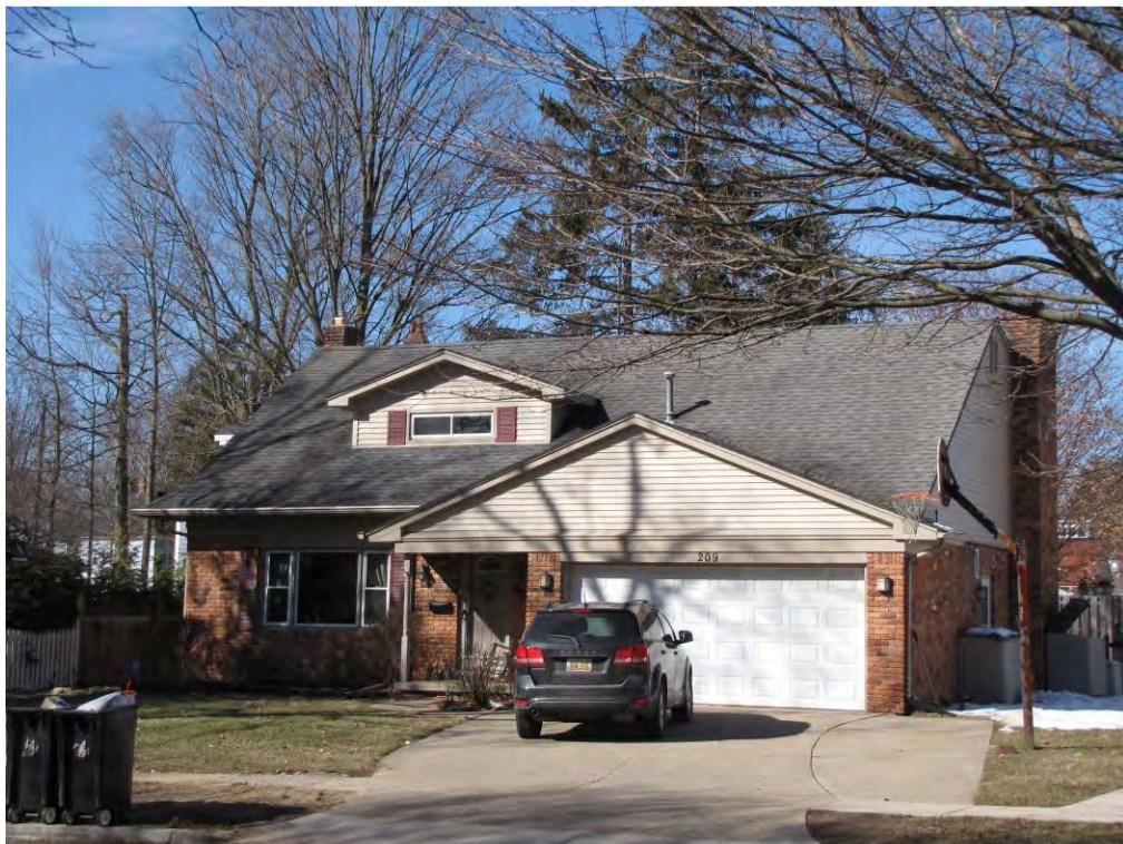
Wing North 209_Looking Southwest
