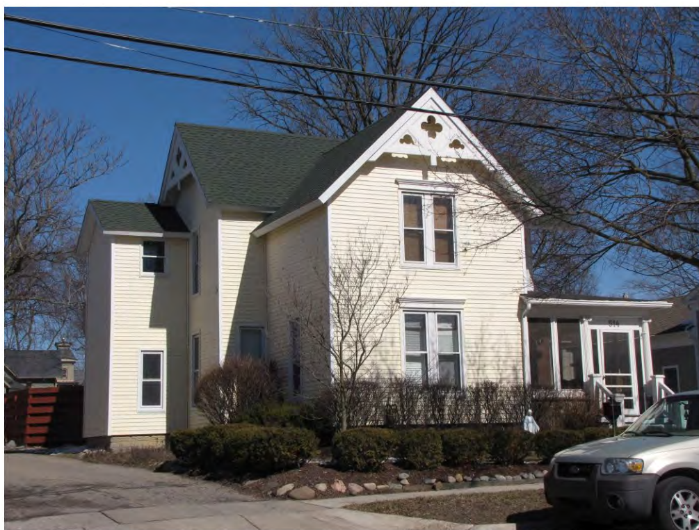
Main West 514_Looking Northeast
