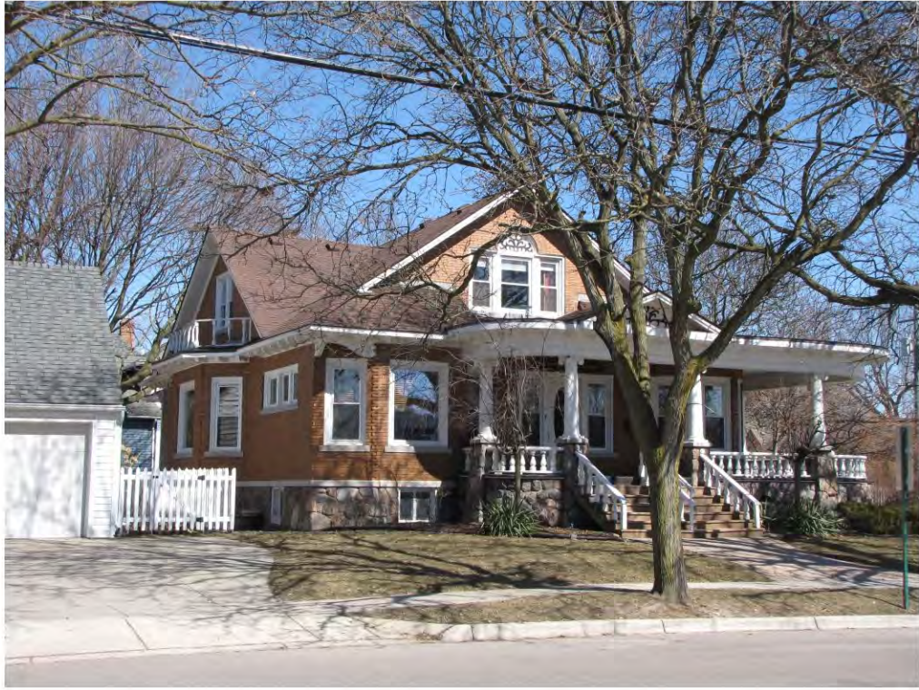
Main West 302_Looking Northeast
