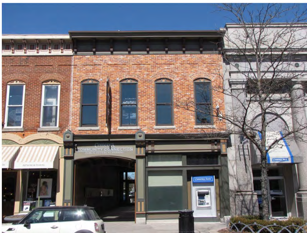
Main East 125_ Looking North
