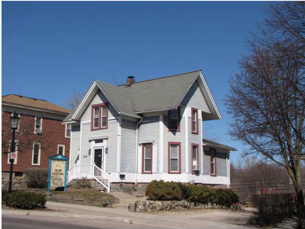
Main East 355_ Looking Northwest
