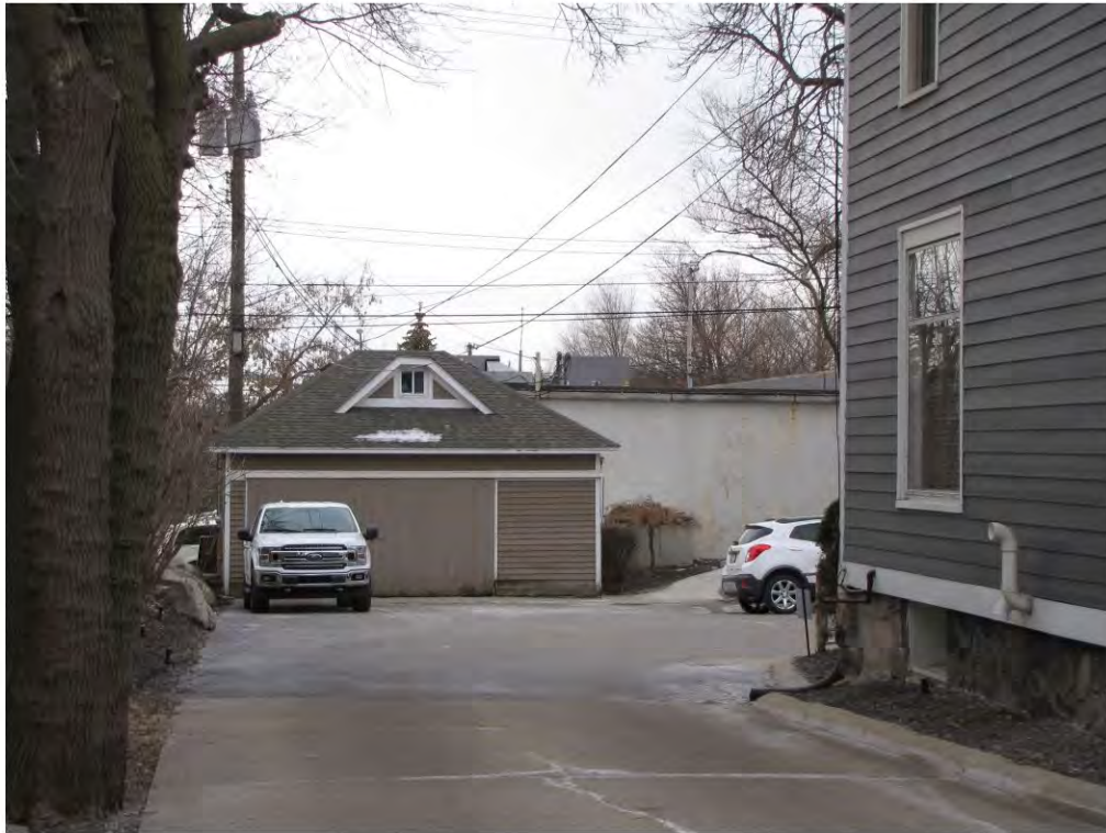
Main East 422, Garage_Looking South
