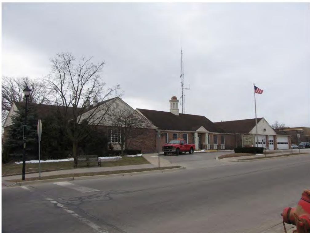
Main West 215_Looking Southwest
