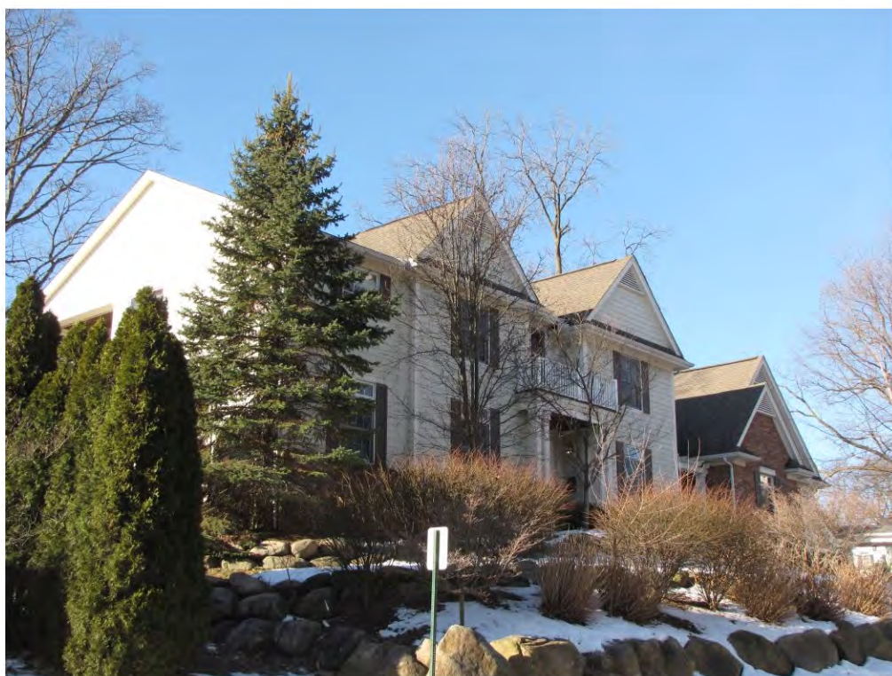
Linden Court 515_Looking Southwest
